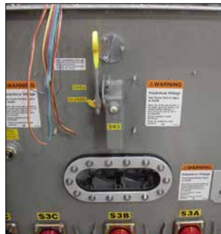
Figure 8. VFI transformer with visible break.
