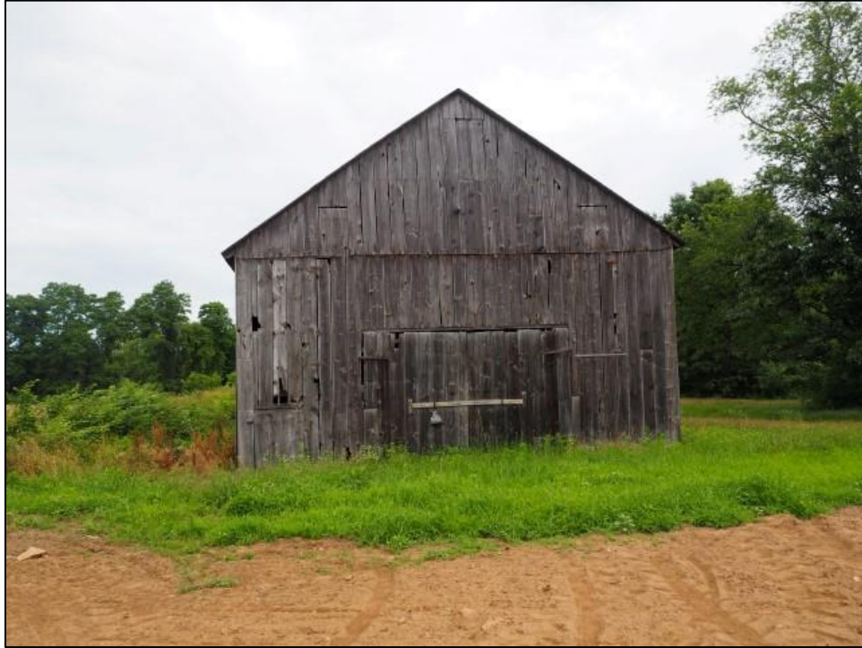
Figure 41. Frontal view of Tobacco Shed No.5 facing southeast.
