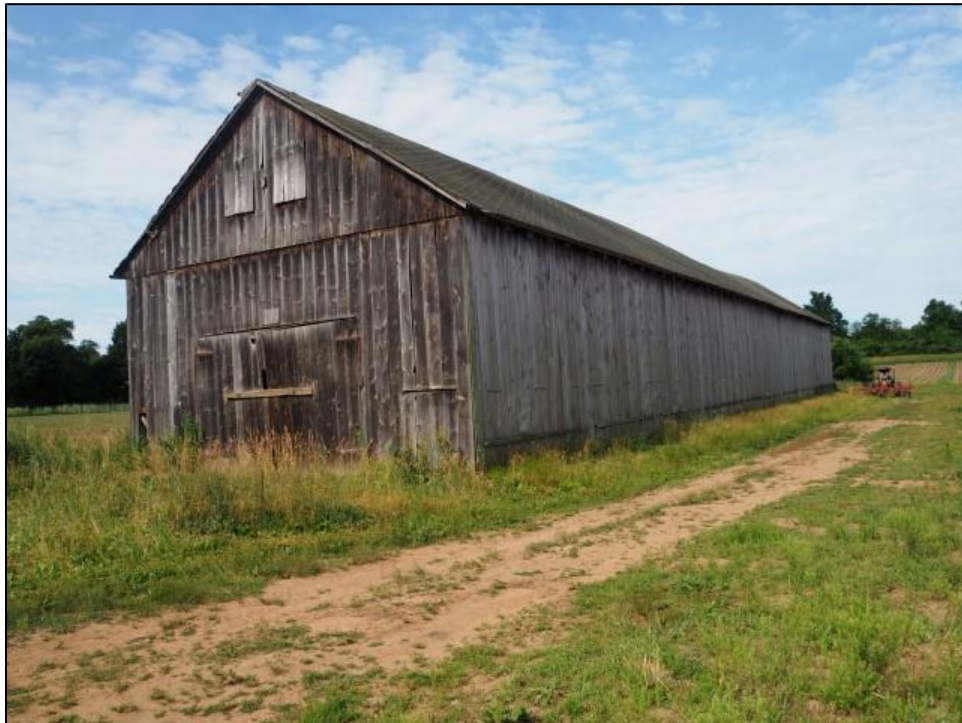
Figure 34. Three-quarter view of Tobacco Shed No.1 facing Barber Hill Road. View is southwest.
