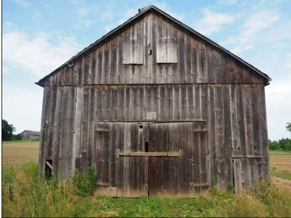
Figure 33. Frontal view of Tobacco Shed No.1 facing Barber Hill Road to the east. View is west.
