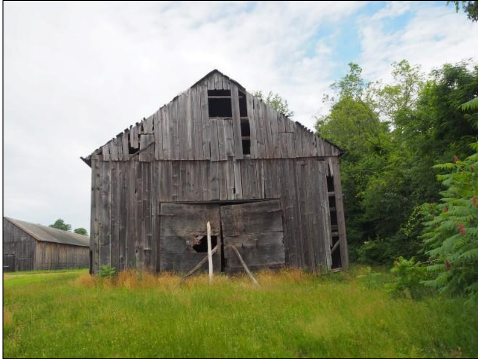
Figure 39. Frontal view of Tobacco Shed No. 4 facing southeast.
