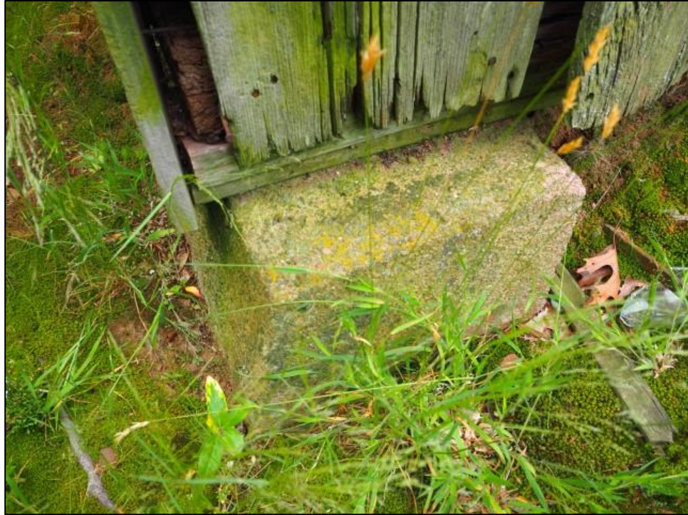
Figure 45. Footing at northeast corner of Tobacco Shed No. 4.
