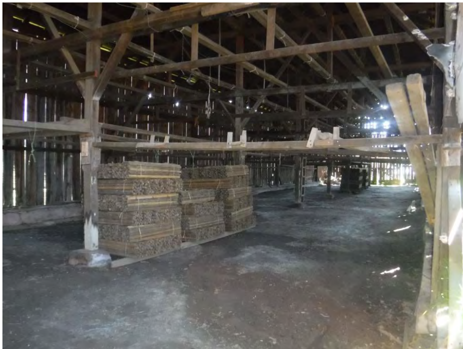
Photograph 10: 029-68-010 - Rockville Rd, inside Barn #3
