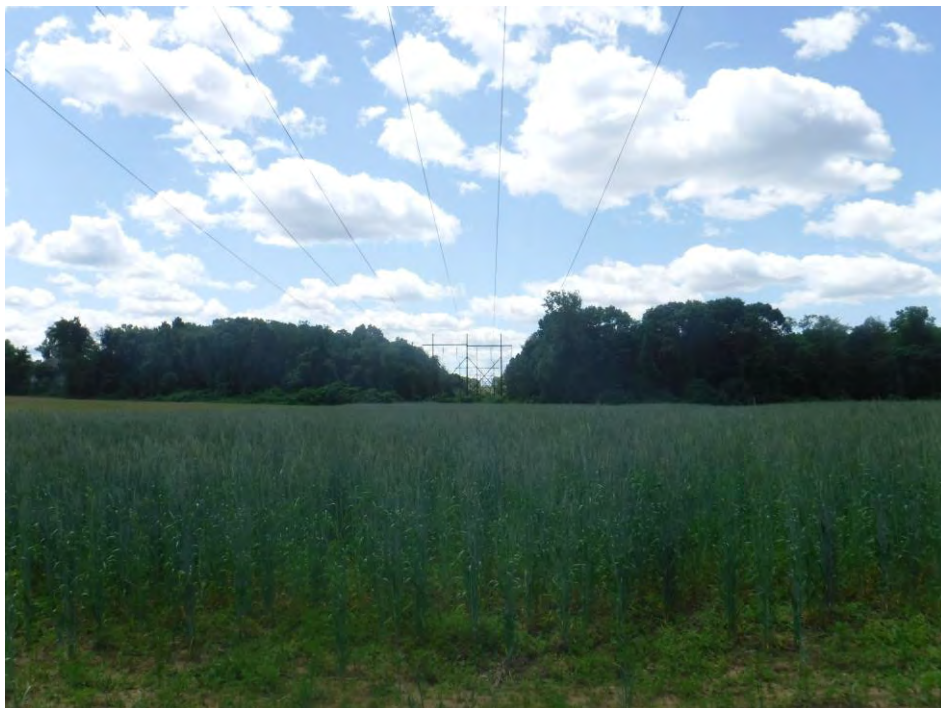
Photograph 20: 028-68-023 – Miller Rd, Electrical lines running north/south
