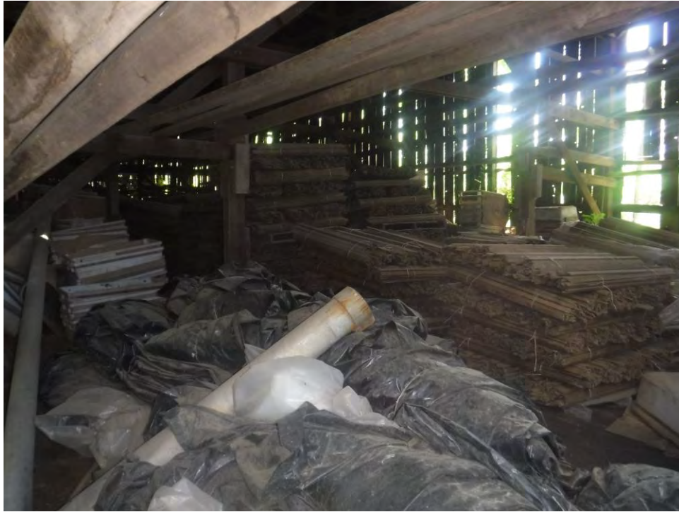
Photograph 21: 028-68-023 – Miller Rd, Inside Barn #5
