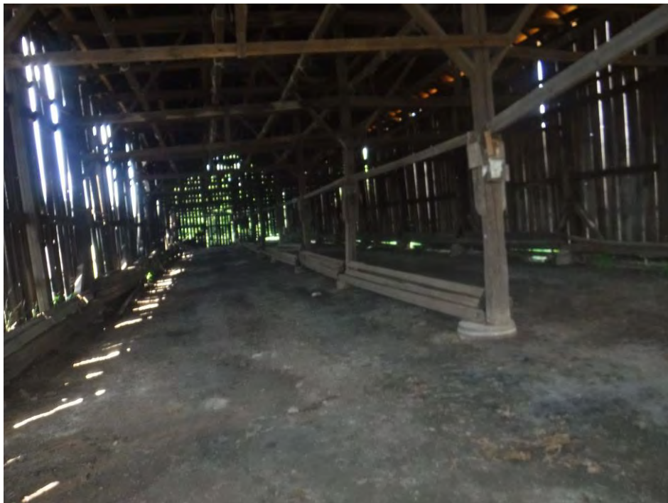
Photograph 22: 028-68-023 – Miller Rd, Inside Barn #6
