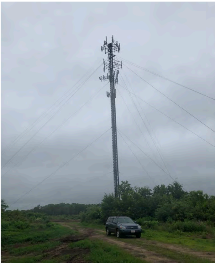
Cell tower, looking west.
