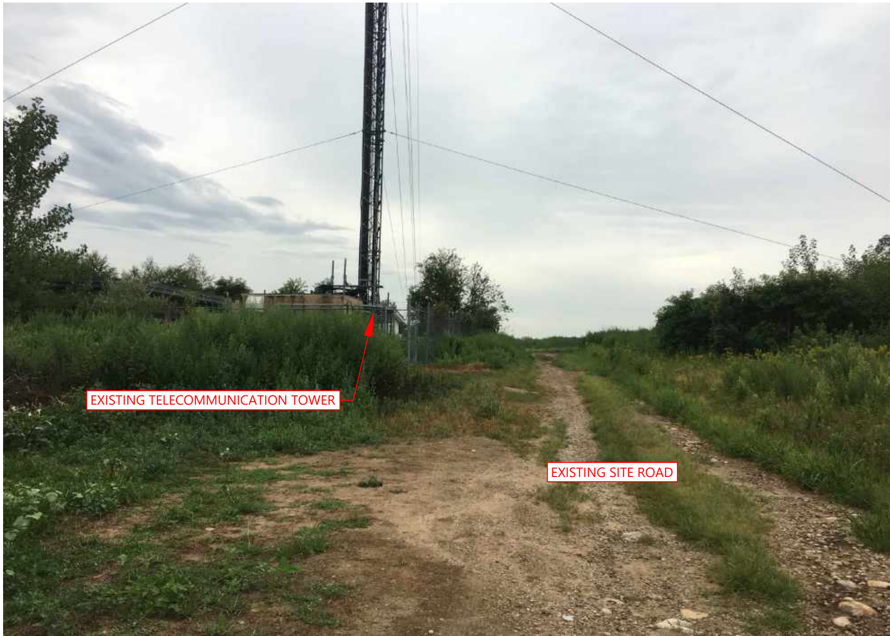
Photo 2 Existing Farm Road To Site Looking North
