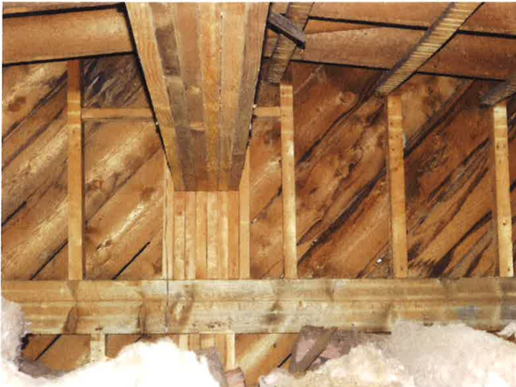
Photo 2: Sample photo illustrating the existing roof construction.
