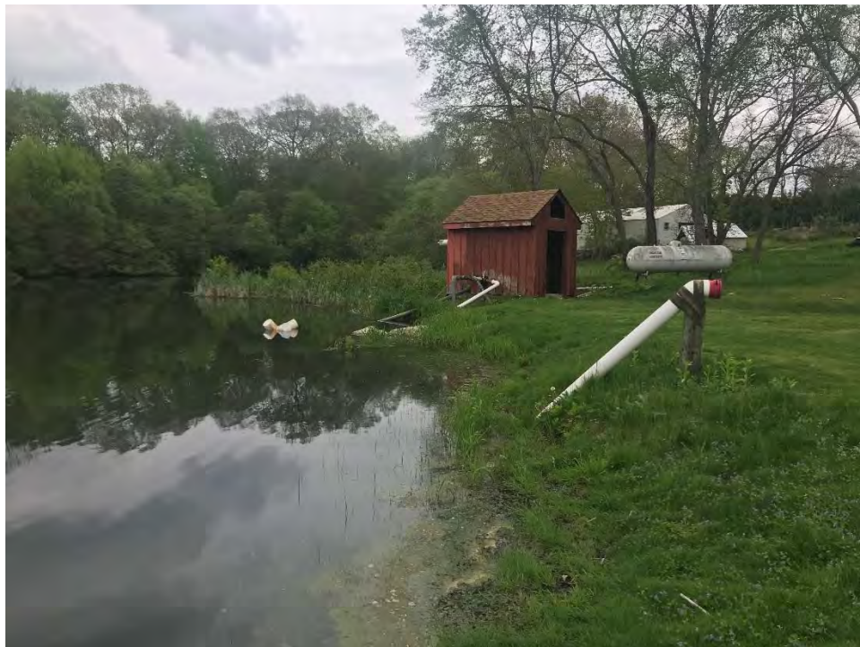
Irrigation Pond Withdrawal Point (Pump 1). Dry Hydrant in Foreground.
