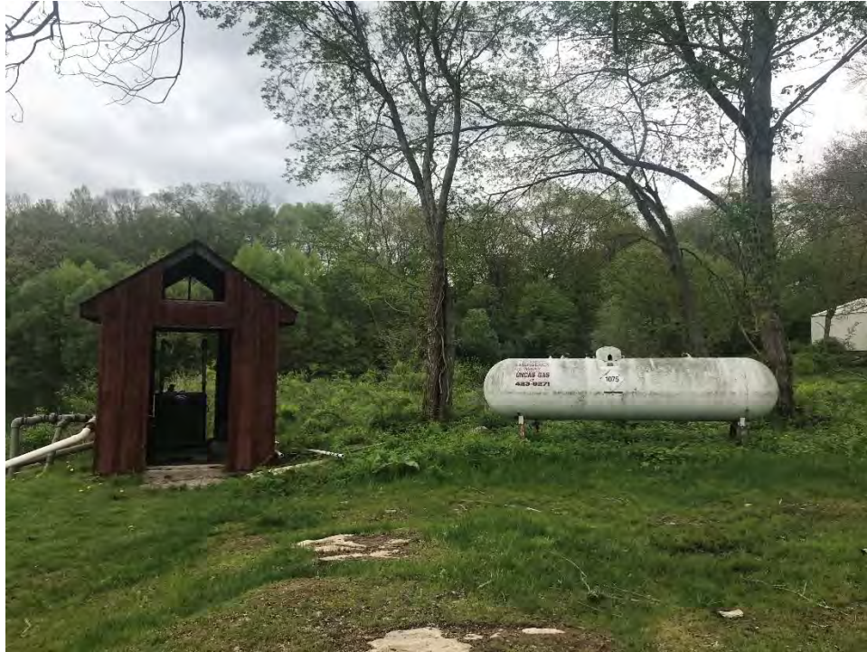
Irrigation Pond Withdrawal Point (Pump 1). Dry Hydrant in Foreground.
