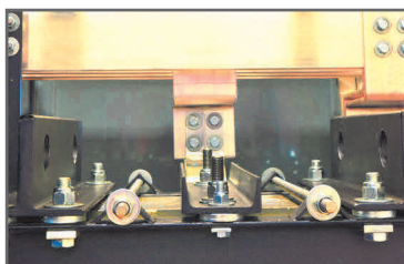
Lifting eyes for core & coil assembly
