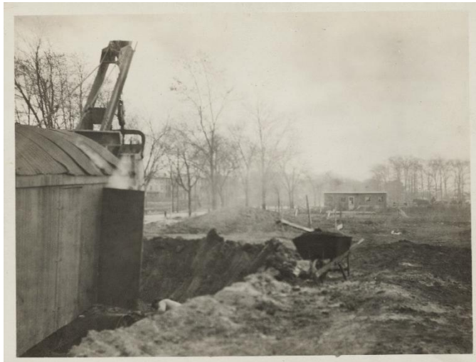
Figure 15 – Excavation of a Basement, Nov. 1918
