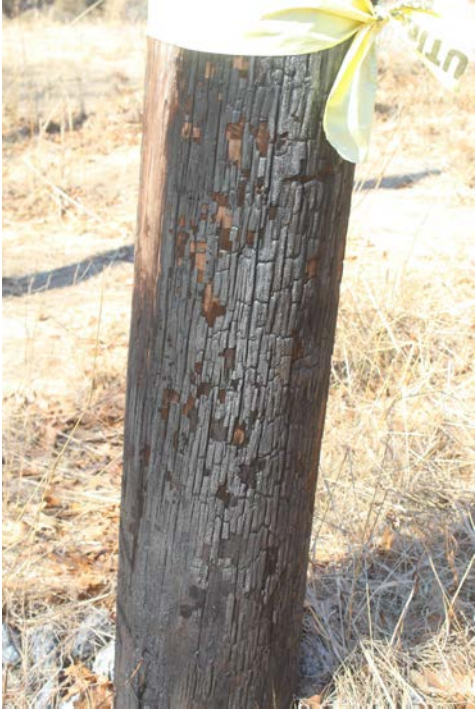
Str. # 8343: Split pole tops, wood pecker damage, cracks, burnt at base.
