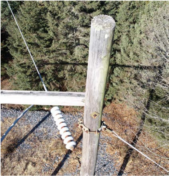
Str. # 8342: Split pole tops, cracks.
