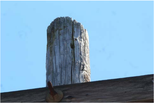
Str. # 8342: Split pole tops, cracks.
