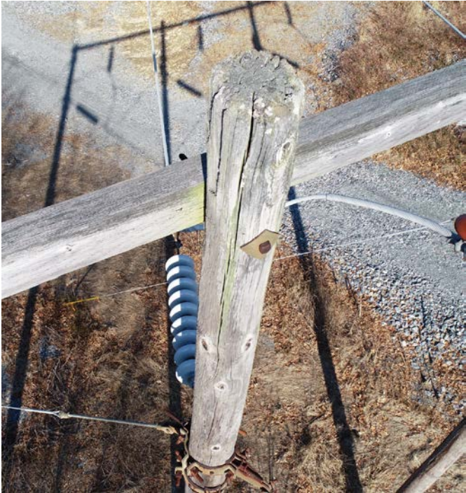
Str. # 8343: Split pole tops, wood pecker damage, cracks, burnt at base.
