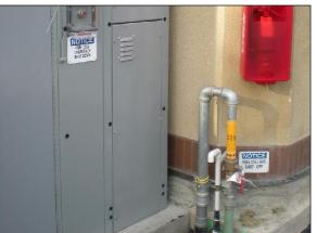
Figure 3: Manual Natural Gas Valve
