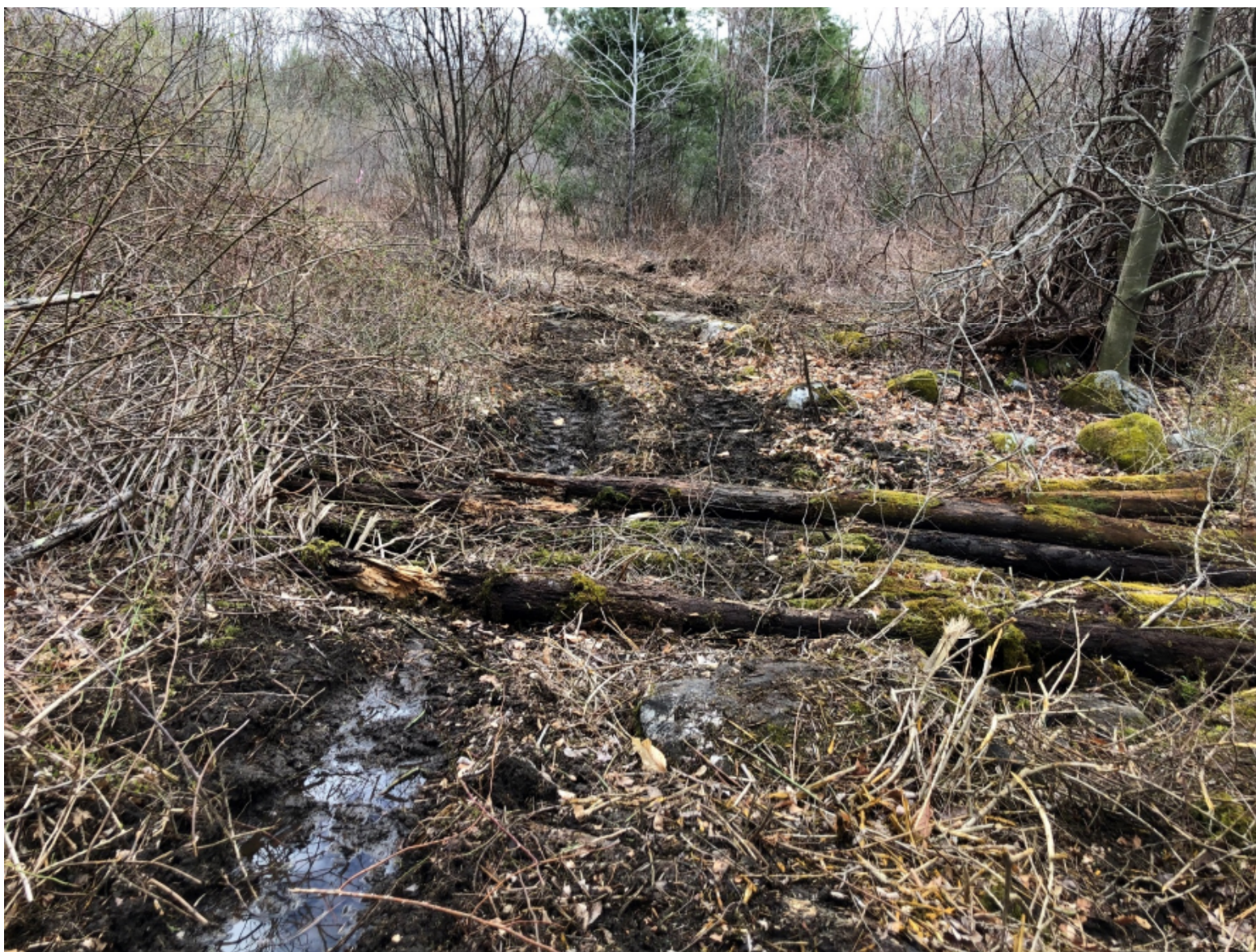
Figure 5 - STANDING ON THE WEST SIDE OF WETLAND CROSSING #1 LOOKING EAST (ORIGINAL CORDUROY CROSSING STILL IN PLACE)
