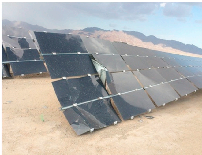
Fig. 4. First Solar's Desert Sunlight section damaged by tornado on July 28, 2015 (source: https://www.ksq.com/news/solar-farm-damaged-by-desert-center-tornado/62923230 ).
