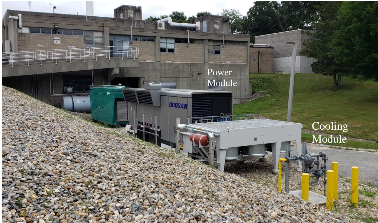
Figure 4. Doosan Fuel Cell Operating at the Montville Site
