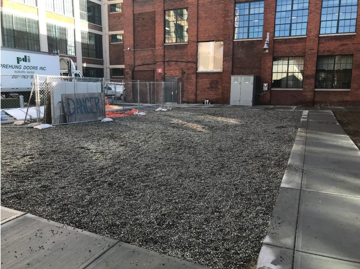
Fuel Cell Area in Courtyard of Cherry St Lofts Attachment #2
