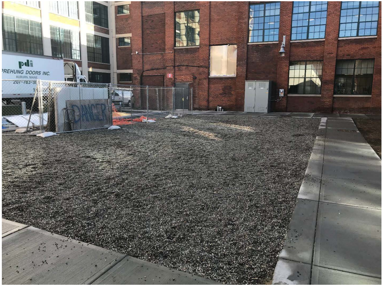
Fig. 2 Picture of the courtyard where the Fuel Cell is to be located
