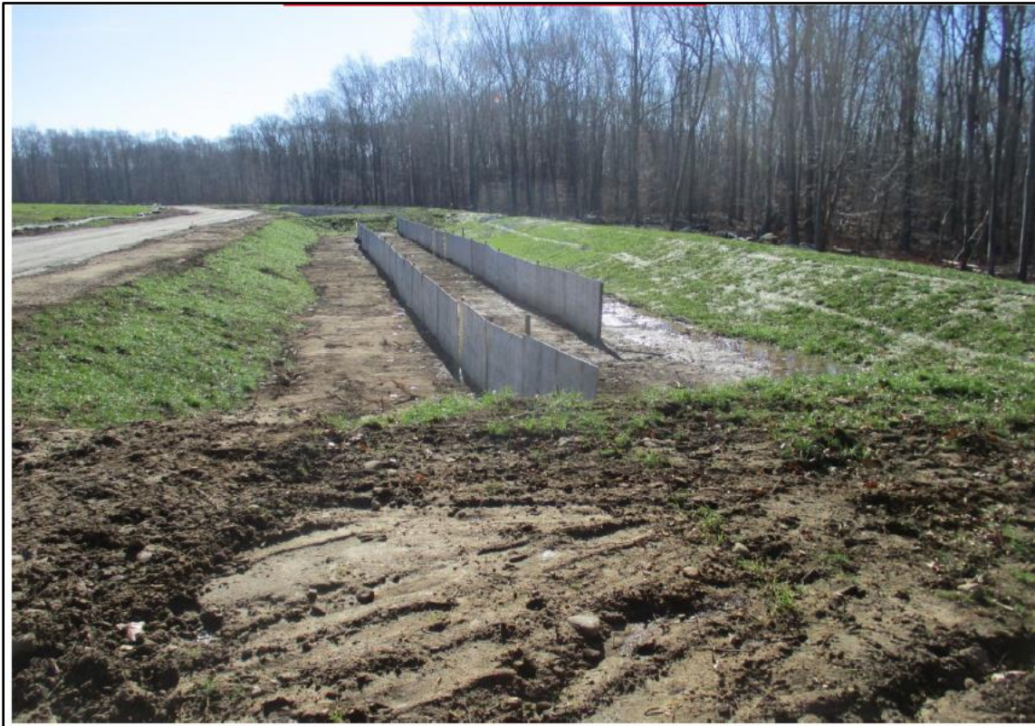
Sediment trap basins with baffles
