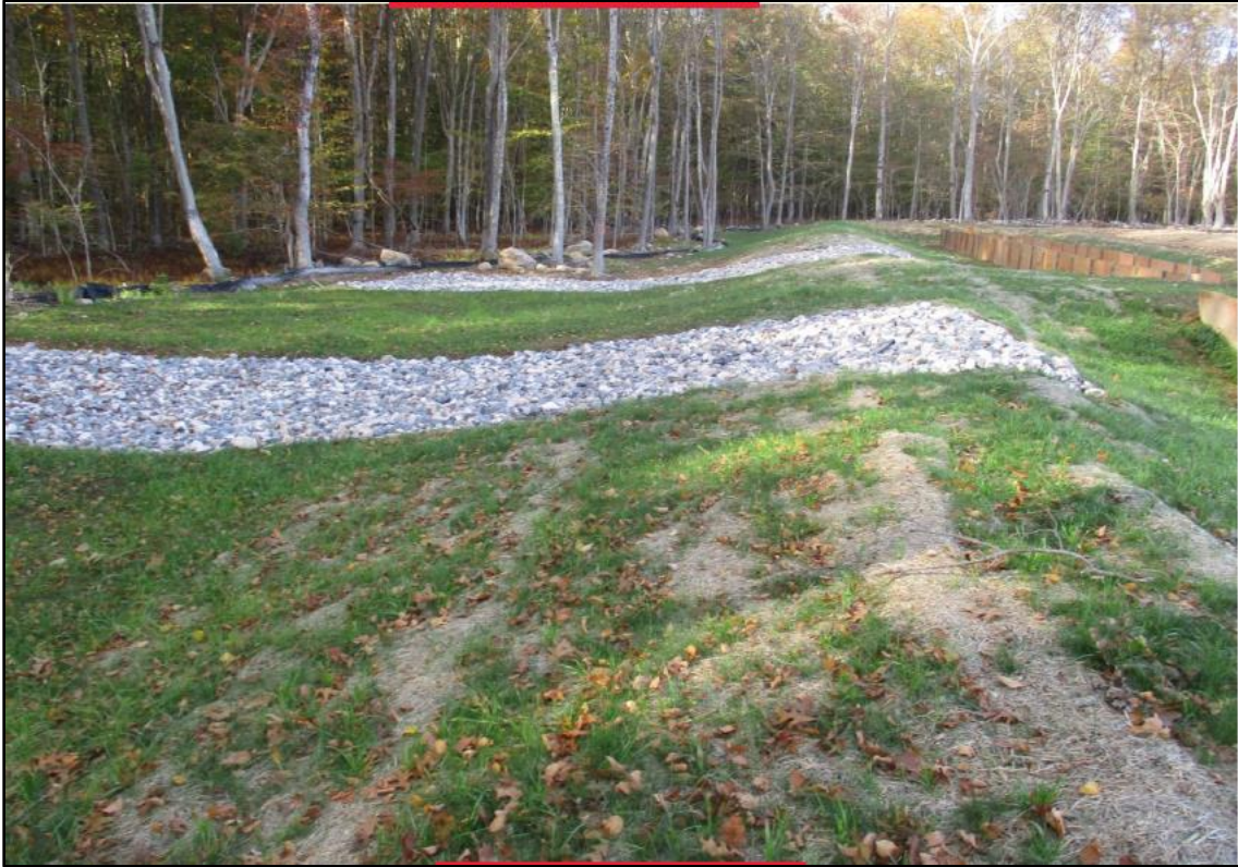
Sediment trap basins with grass growth and stabilization
