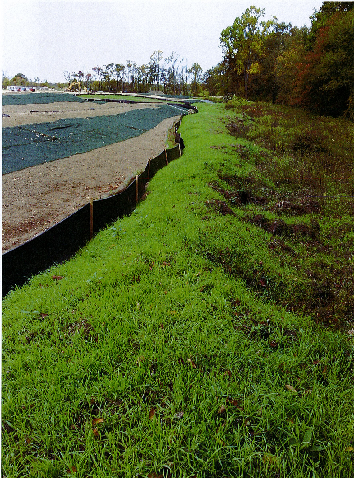
Vegetated berm. Leaky berm with geotext fabric. To upper left. Phase 1.
