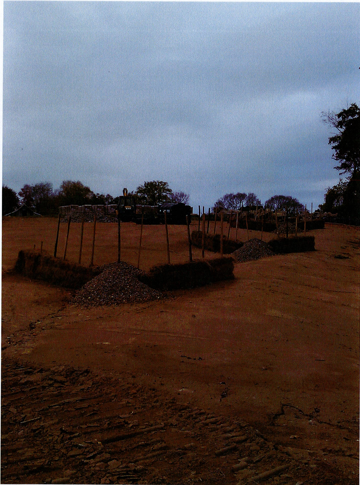
Sediment check dams. Phase 1. Racking system stored on-site beyond excavator.
