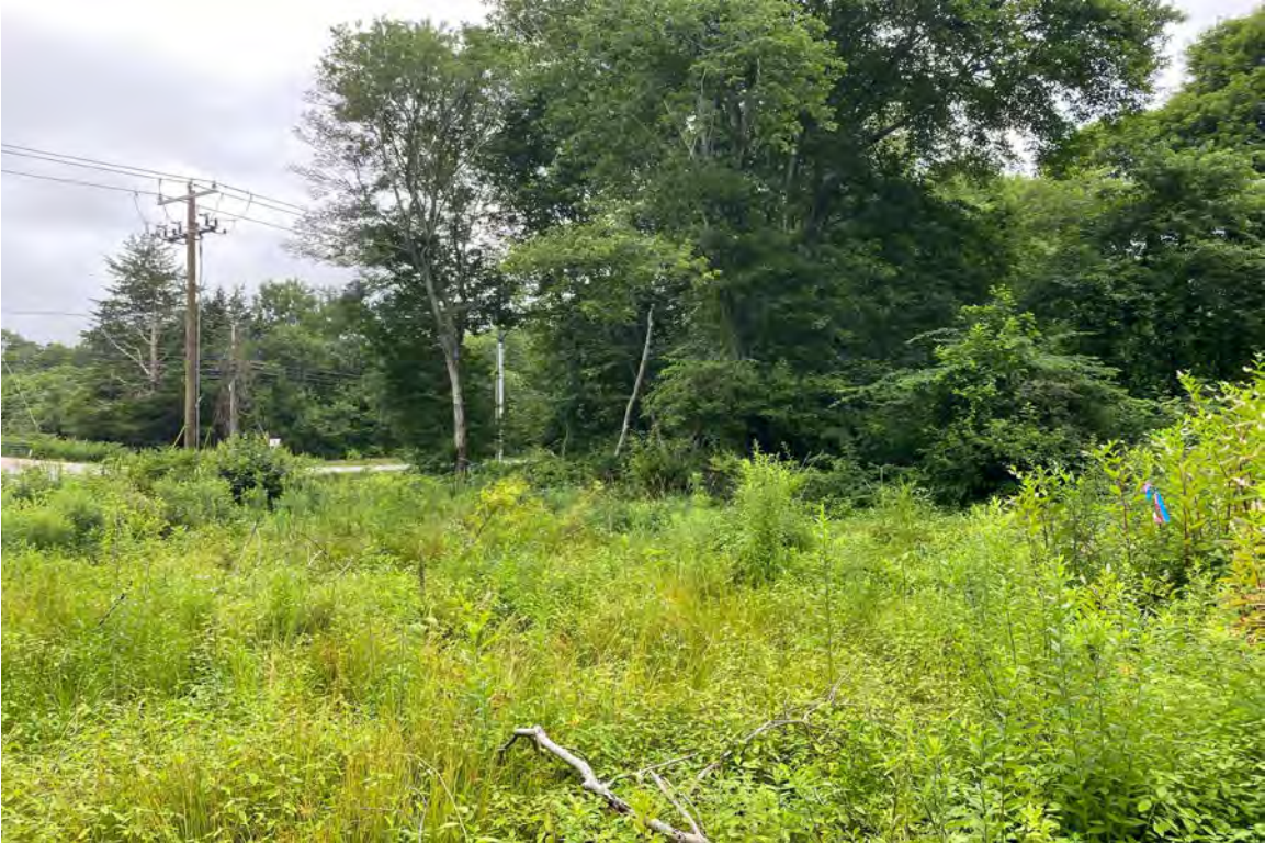
Photo 1: View of proposed wetland crossing for utility interconnection maintenance road looking northwest. Pendleton Hill Road (Route 49) and substation entrance located in left side of photo.
