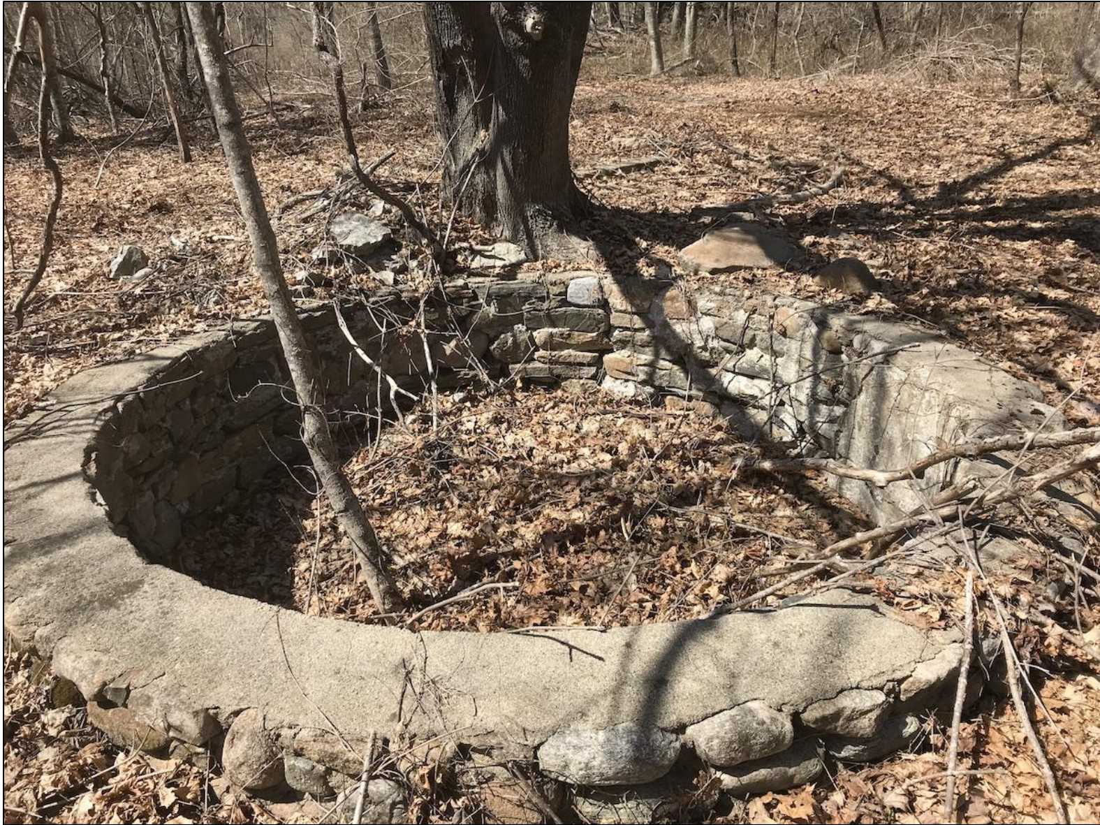
Figure 65. Overview photo of round foundation covered with cement in Area 20.
