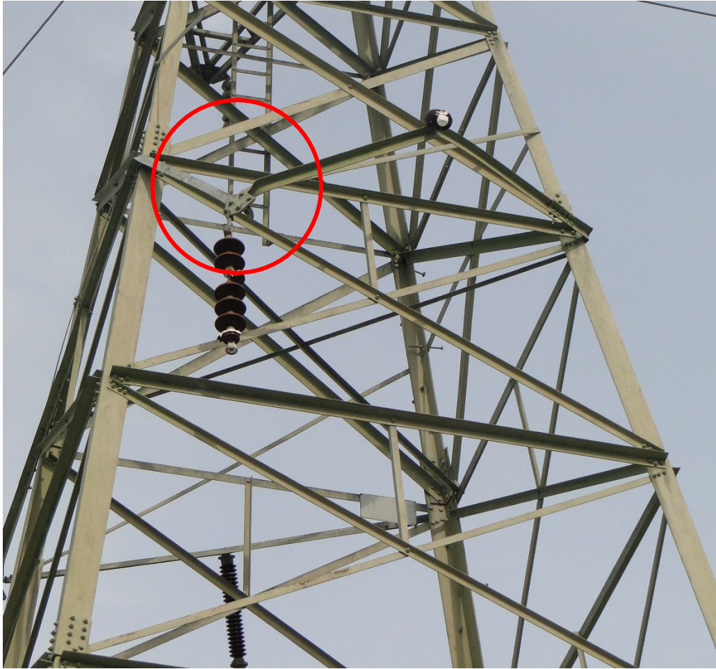
STR 6209 – Another view of arm failure
