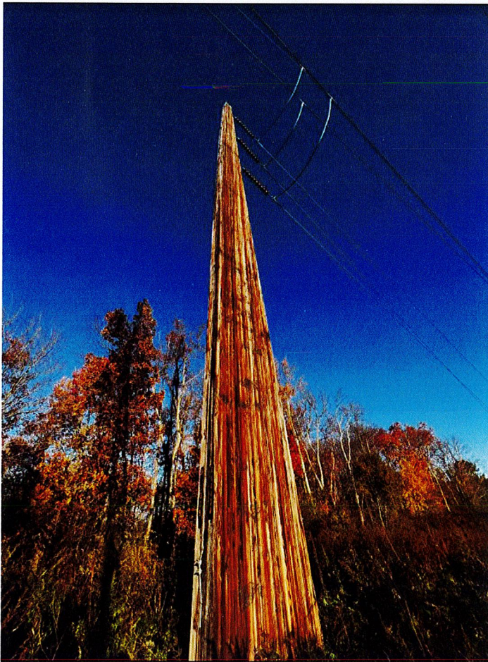
Figure 1: Line 1319 – Existing LWS Structure 1443
