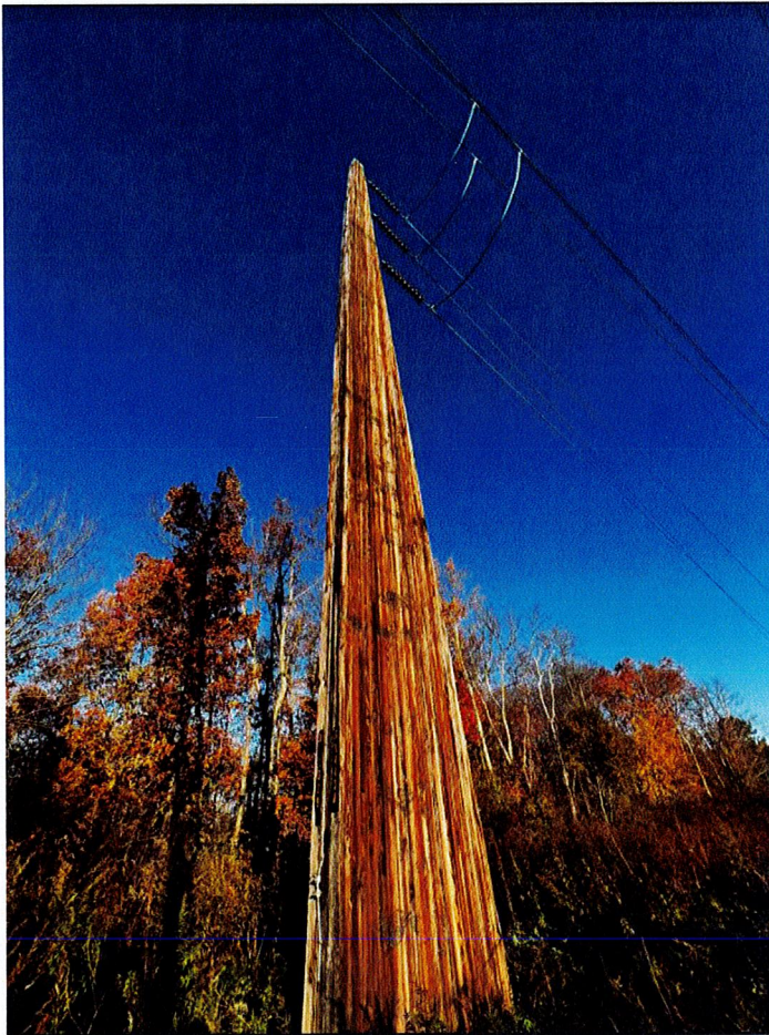
Figure 1: Line 1319 – Existing LWS Structure 1443
