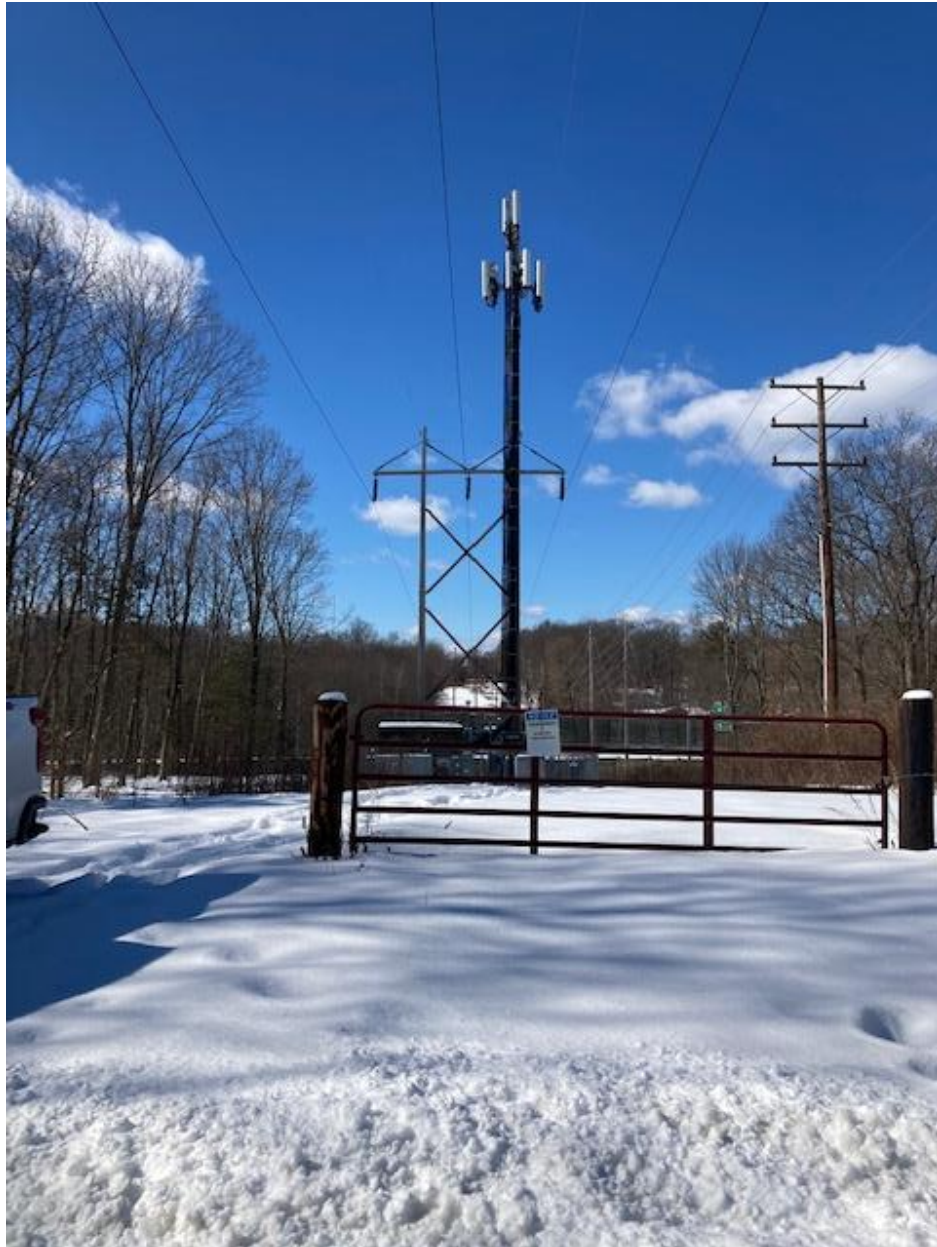
Structure 8012 looking west
