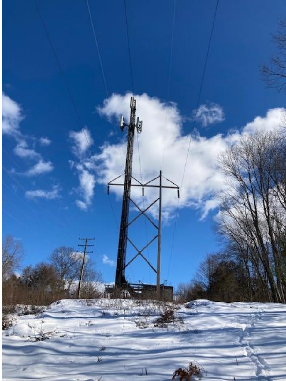
Structure 8011 Looking East
