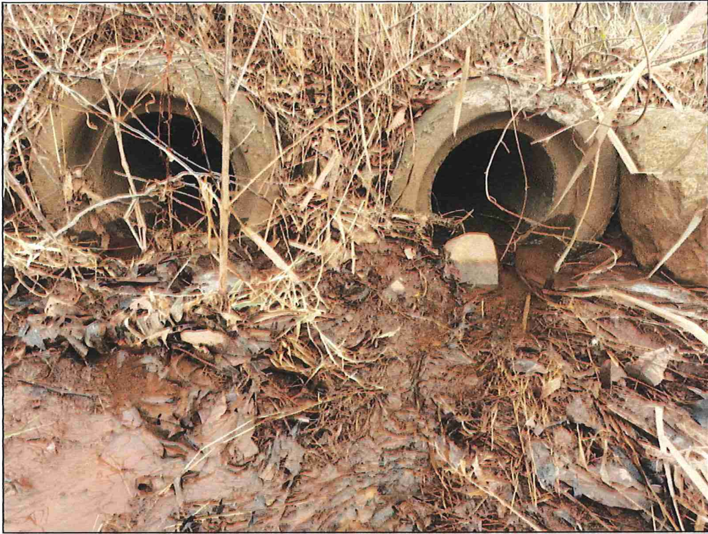
Photo 5. Twin outlet pipes through the "pond" embankment (berm); facing northerly
