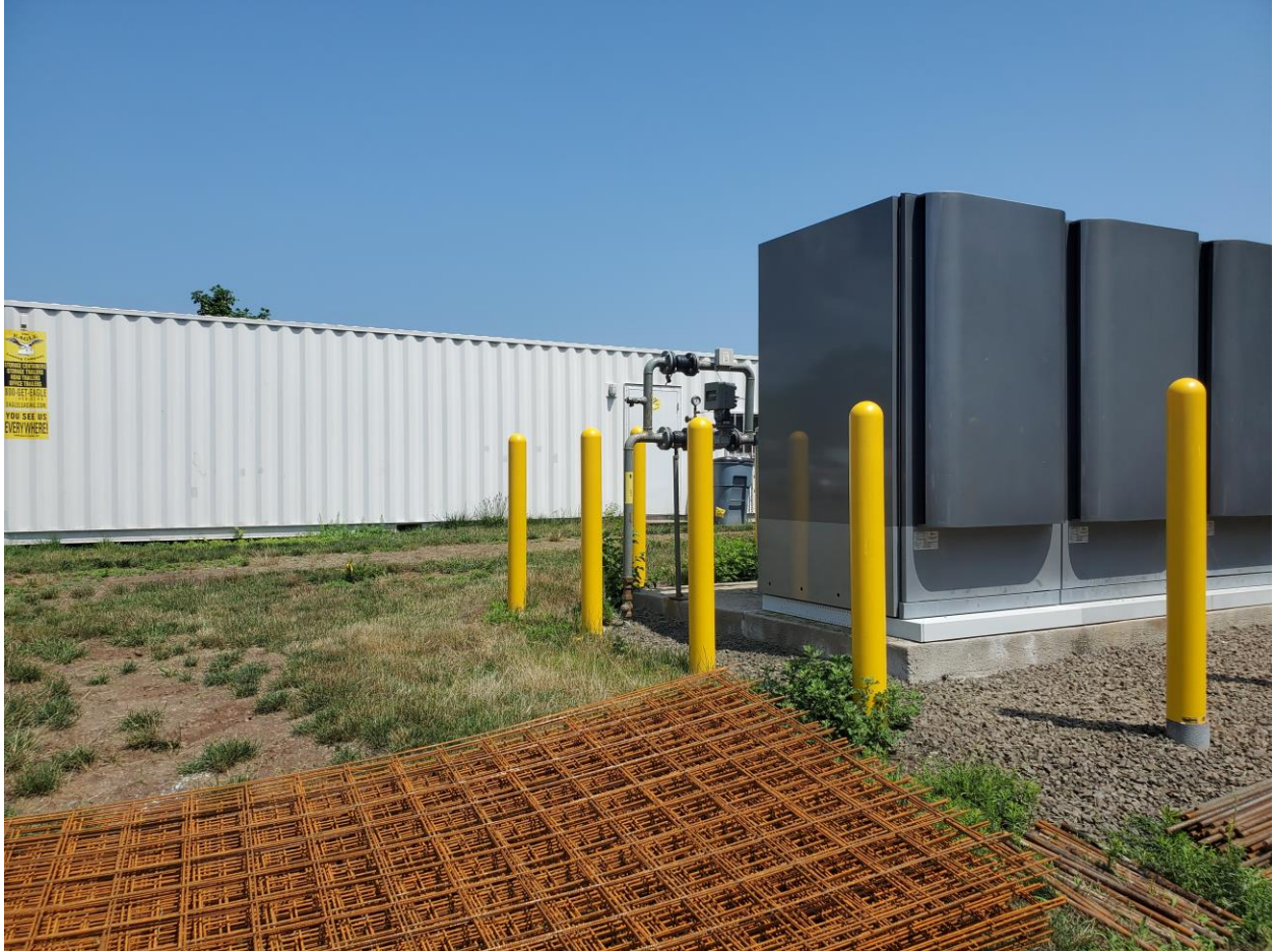
Looking east to location of proposed installation
