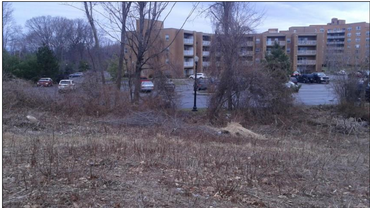
Photo 10. Overview photo of the area to the west of the Mix Avenue Substation facing north (note disturbed areas and debris in this area).
