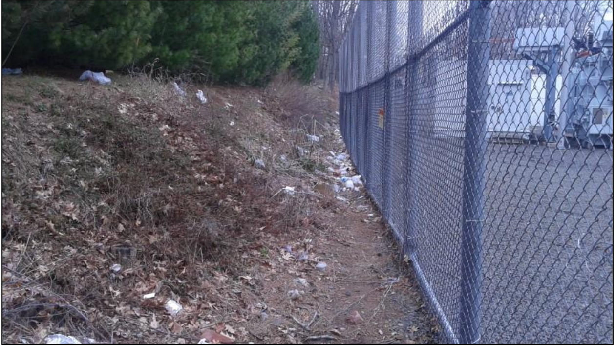
Photo 5. Overview photo of the area to the north of the Mix Avenue Substation facing east.
