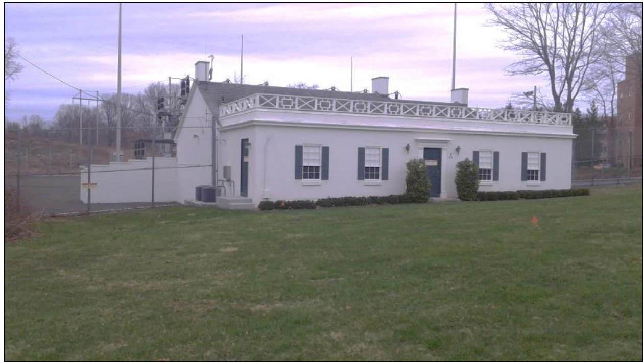
Photo 2. Overview photo of the existing Mix Avenue Substation facing northwest.
