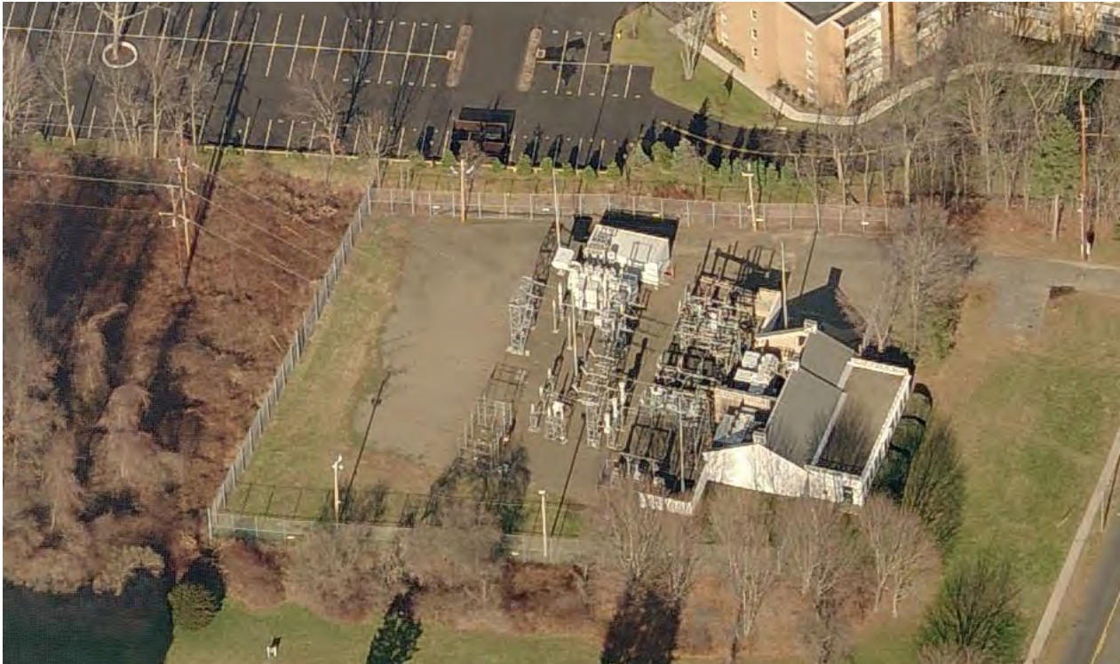
Figure A. Mix Avenue Substation - Existing
