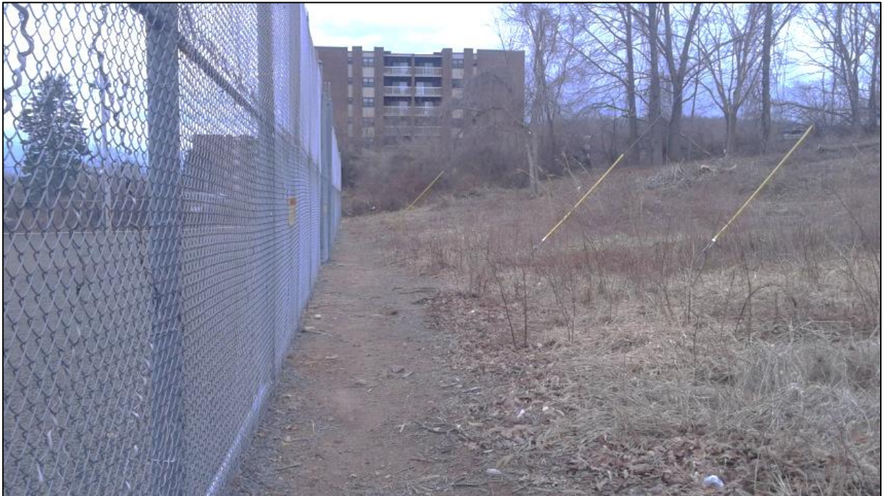
Photo 4. Overview photo of the area to the west of the Mix Avenue Substation facing south.
