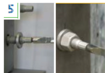
5 Slide the face washer forward and move the nut up to fasten to the bolt. Tighten the nut snug tight at this point.
