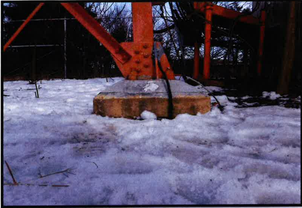
5) VIEW OF FOUNDATION AT GROUND SURFACE
