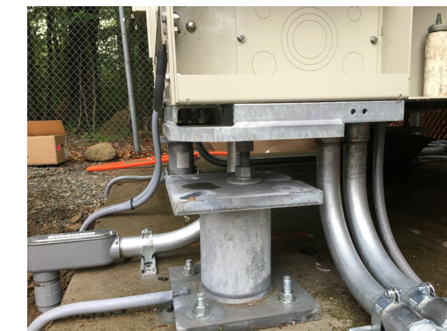
TYP. FOUNDATION WIC BASE ATTACHMENT KIT
