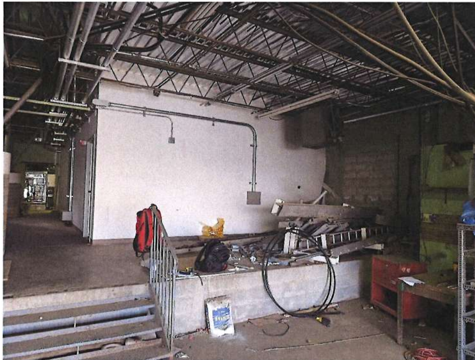
Photo 2: Sample photo illustrating the existing roof framing.
