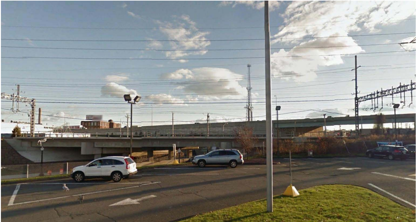
Figure 3: Measurement Location 1 (McDonald's, State Street Extension)
