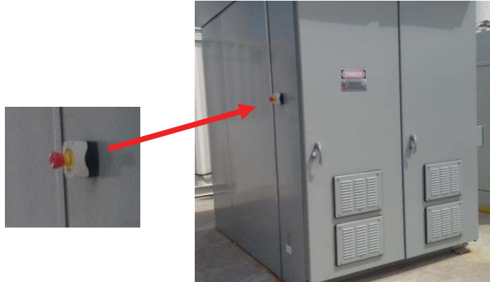
Tie Breaker Switchgear ( Site Electrical Disconnect )
