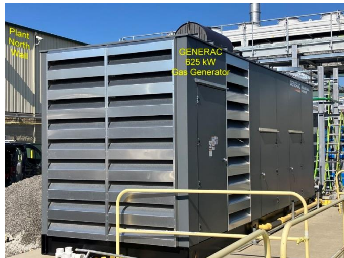
Facility Backup Generator (Existing Source)
