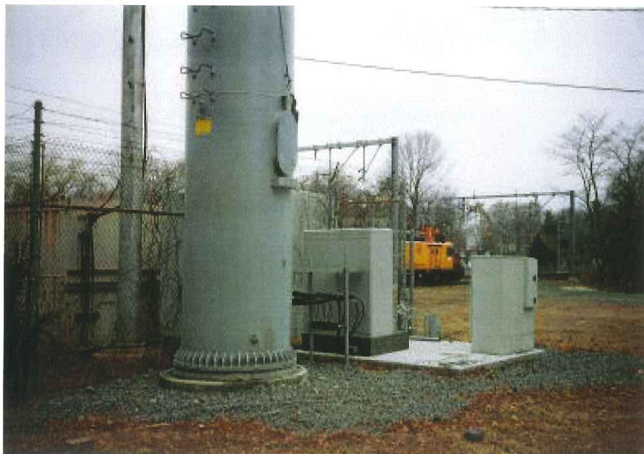
View from the tower looking northeast.
