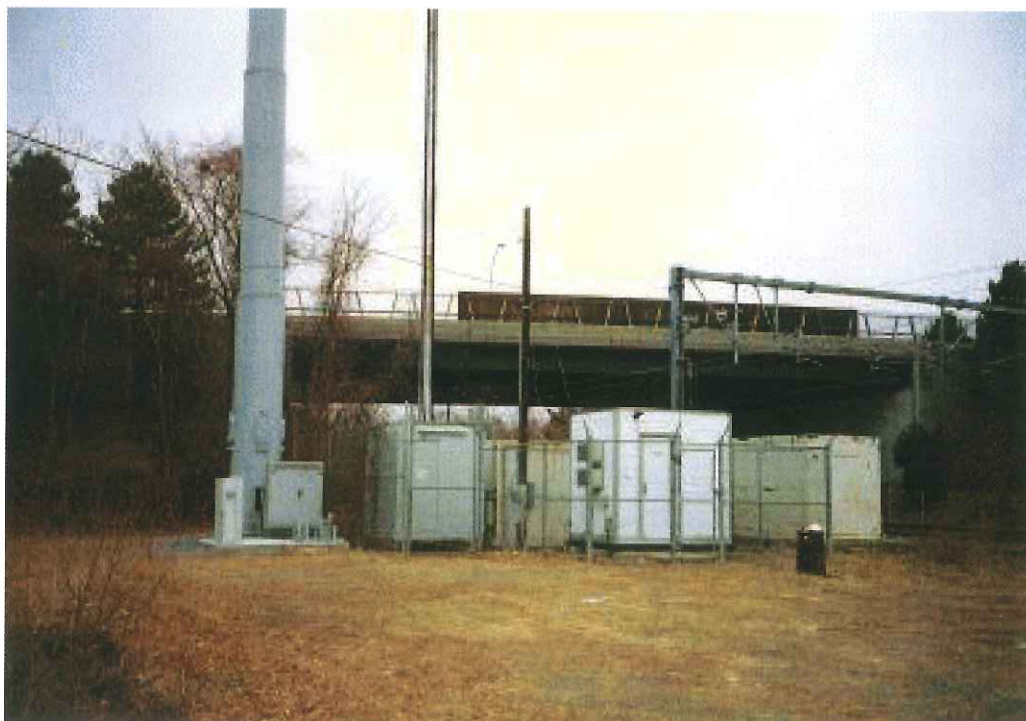
View of the equipment compound looking to the west. The Route One overpass is in the background and the old Amtrak tower is visible to the right of the new monopole. The Railroad tracks are to the north under the catenary structure.
