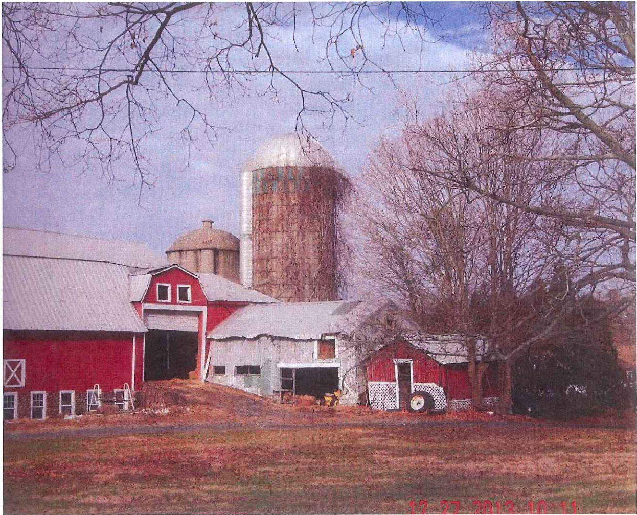
Existing conditions with the (taller) silo proposed to be replaced
