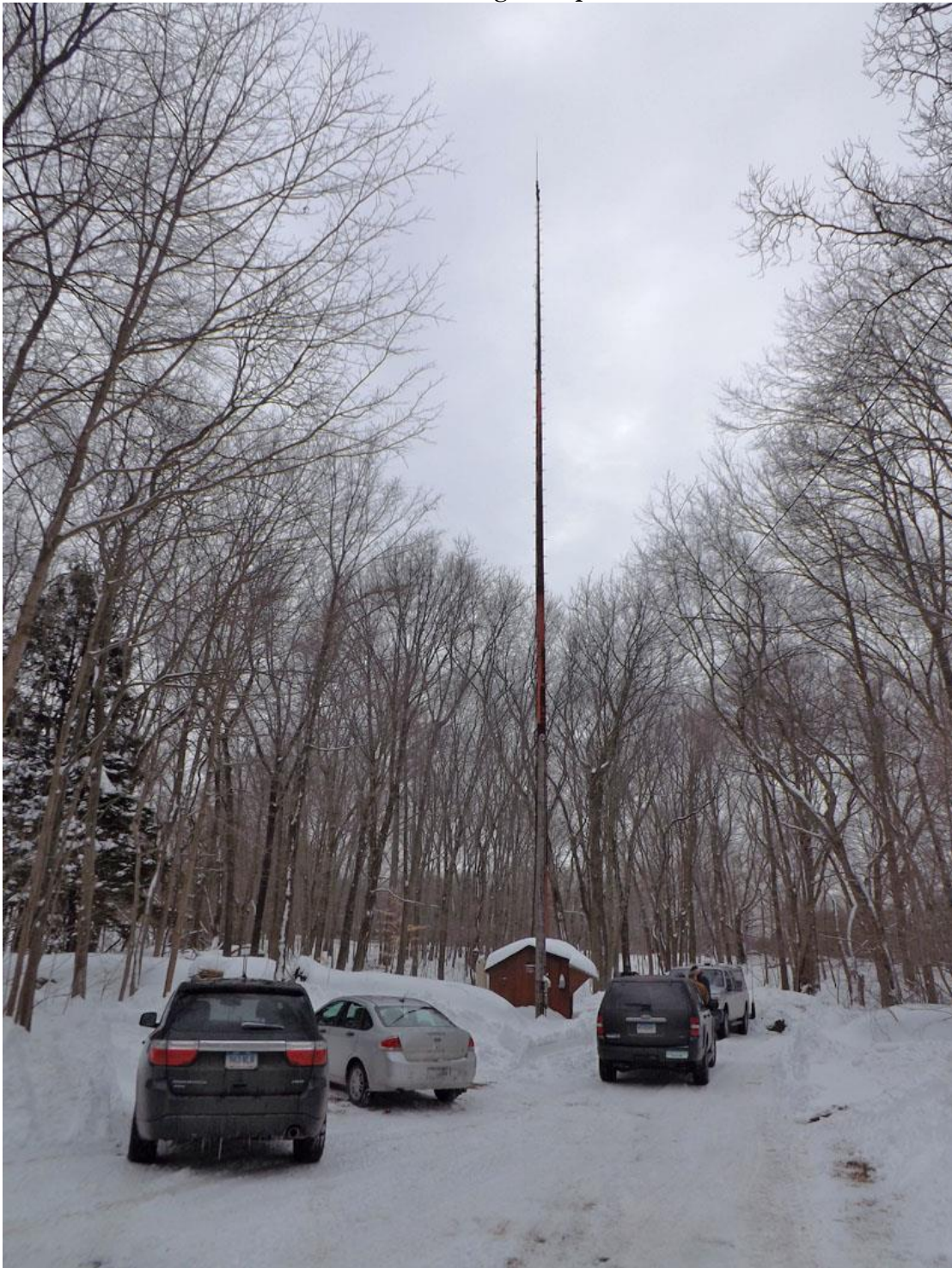
View of existing monopole
