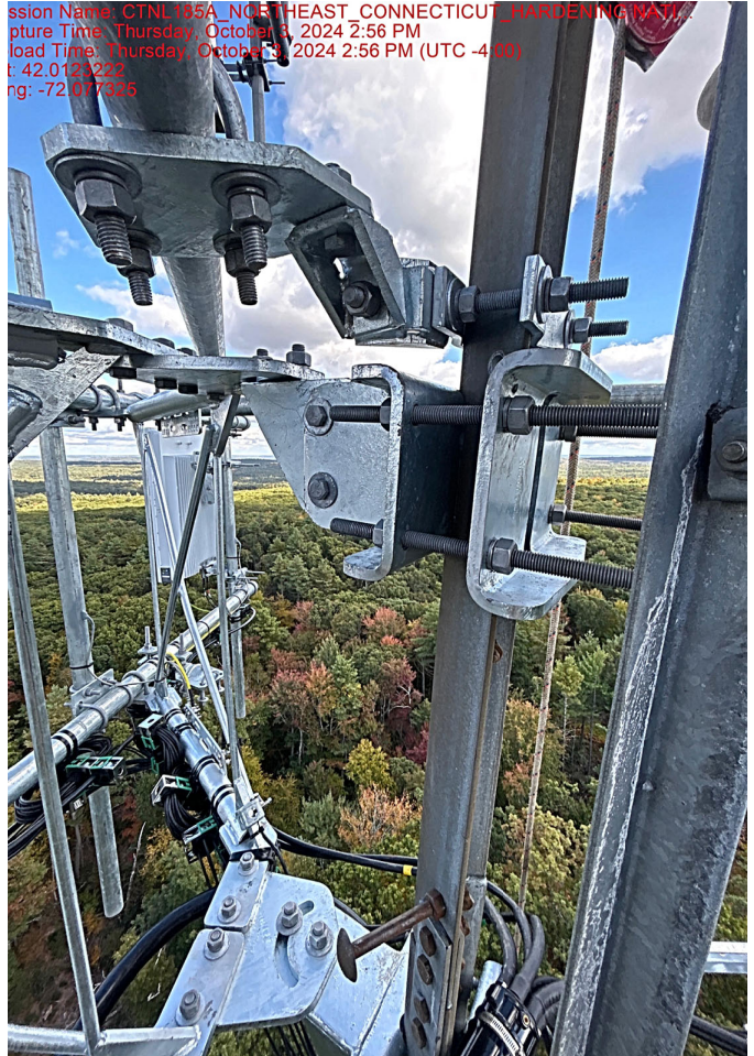
Typical sector frame attachment to tower leg
