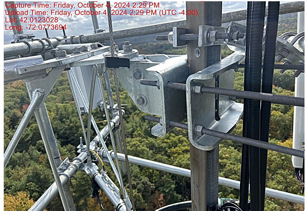
Typical sector frame attachment to tower
