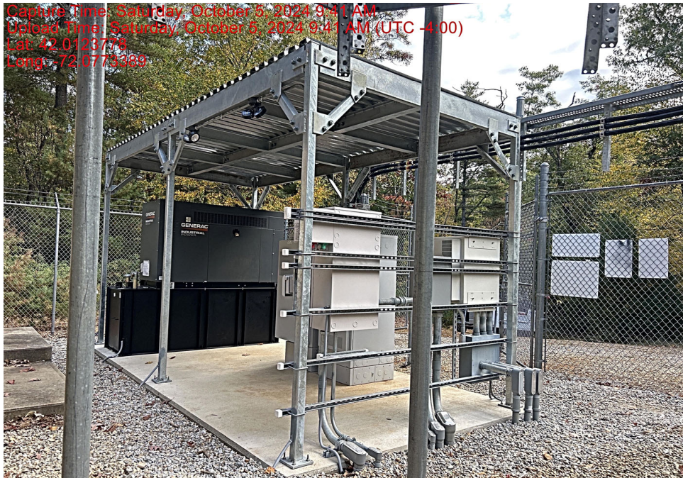
Overall view of new equipment installation
