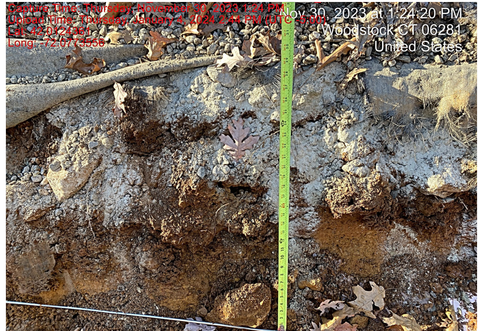
New ground installation
