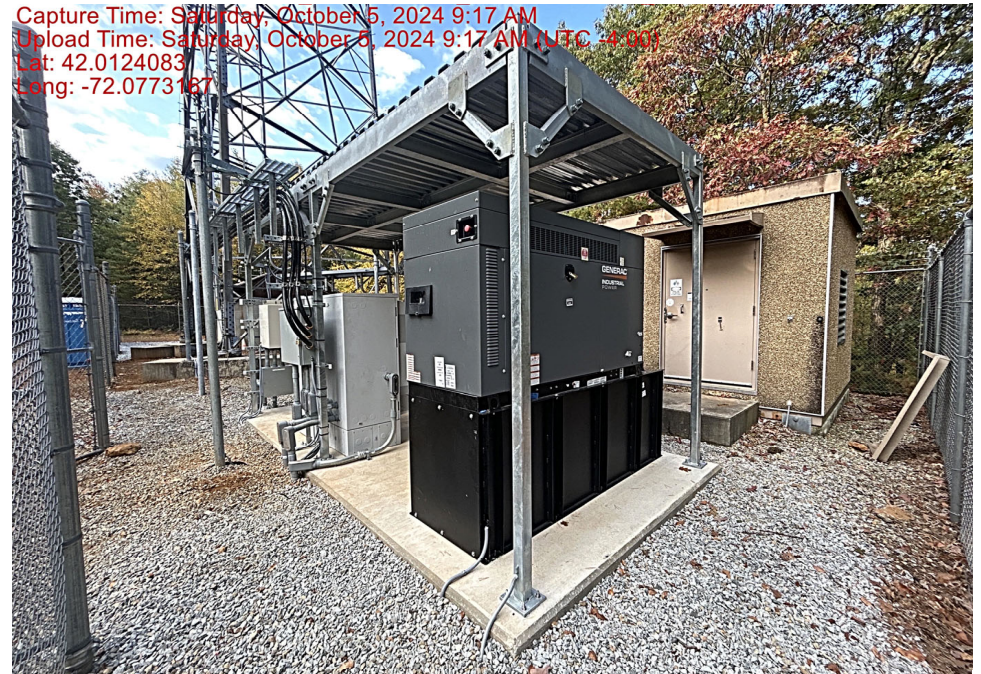
Overall view of new equipment installation
