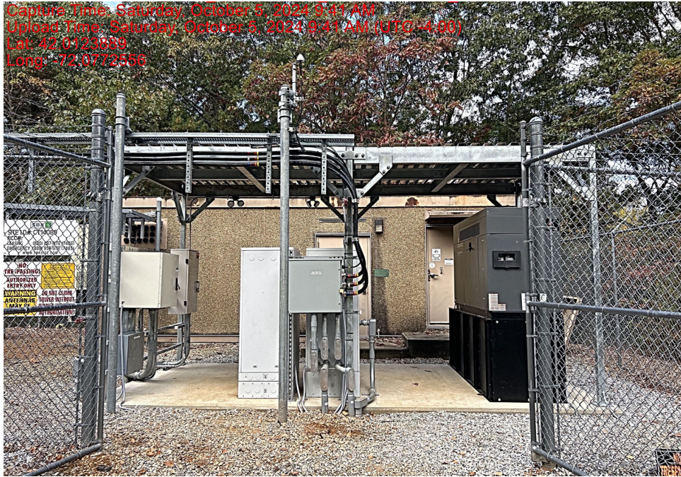
Overall view of new equipment installation
