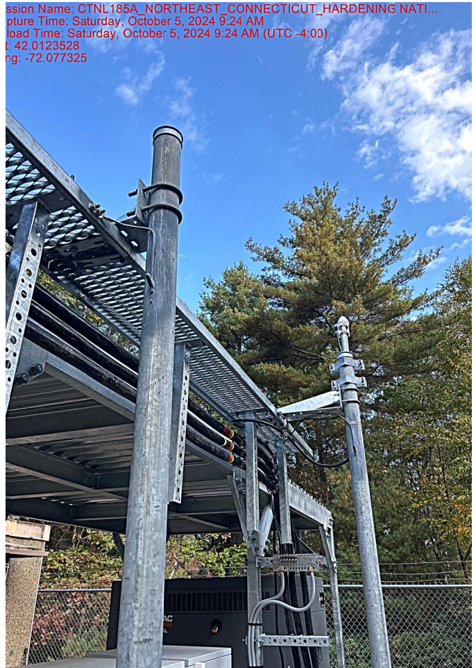
New ice bridge
