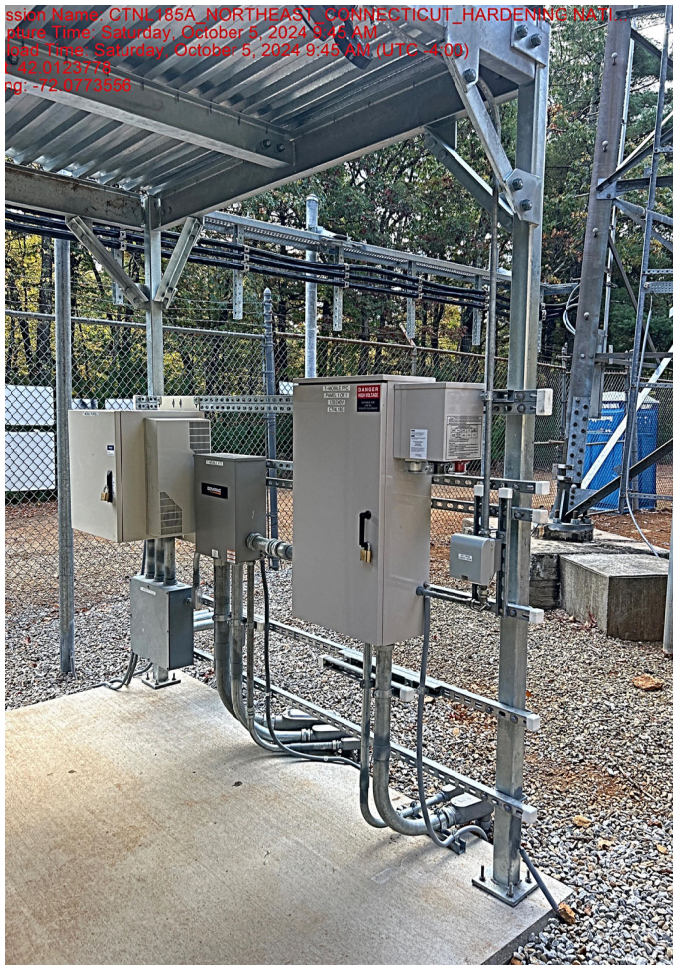
New H-frame for electric and fiber
