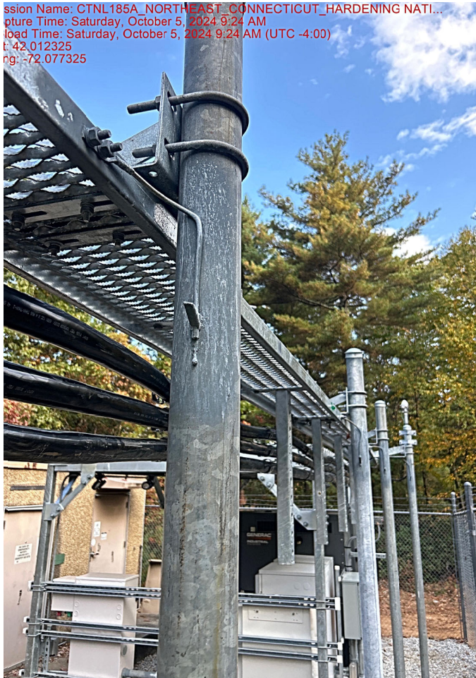
Typical ice bridge installation
