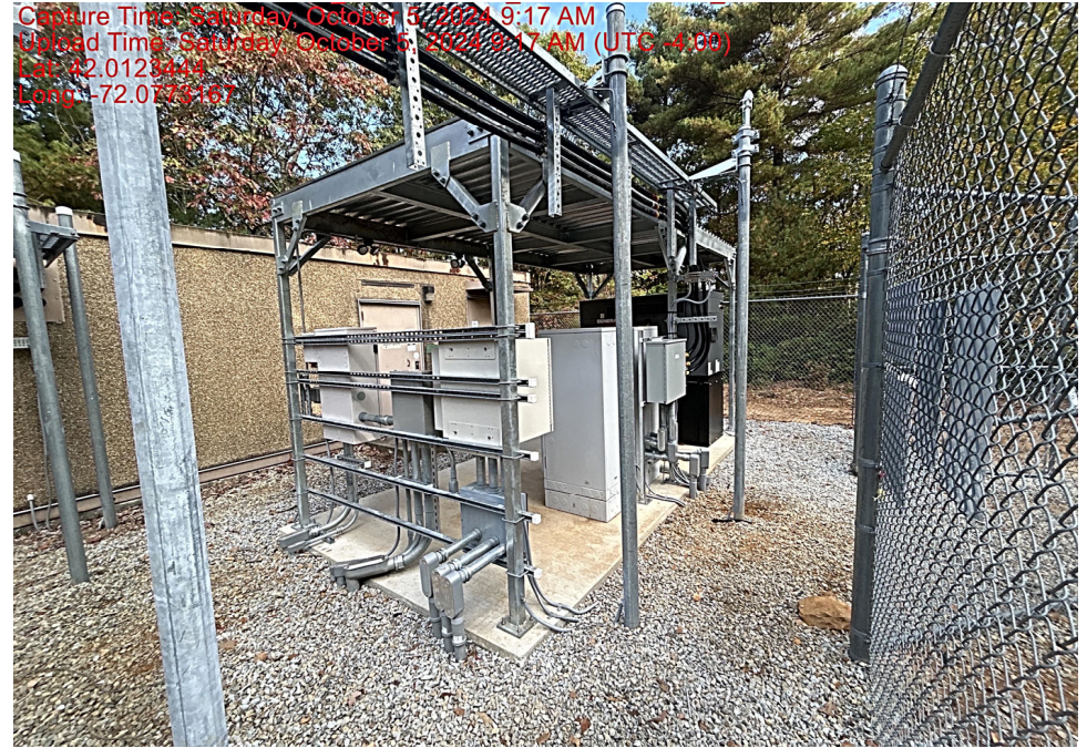
Overall view of new equipment installation
