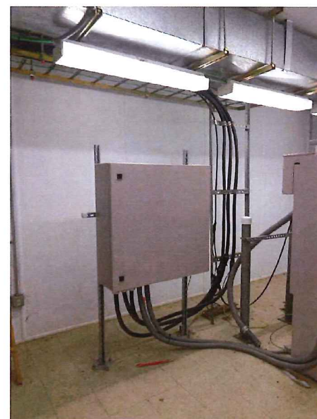
4 EXIST FIBER DISTRIBUTION BOX A-3 SCALE: NTS
