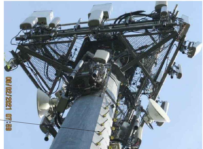
Existing Climbing Facility
