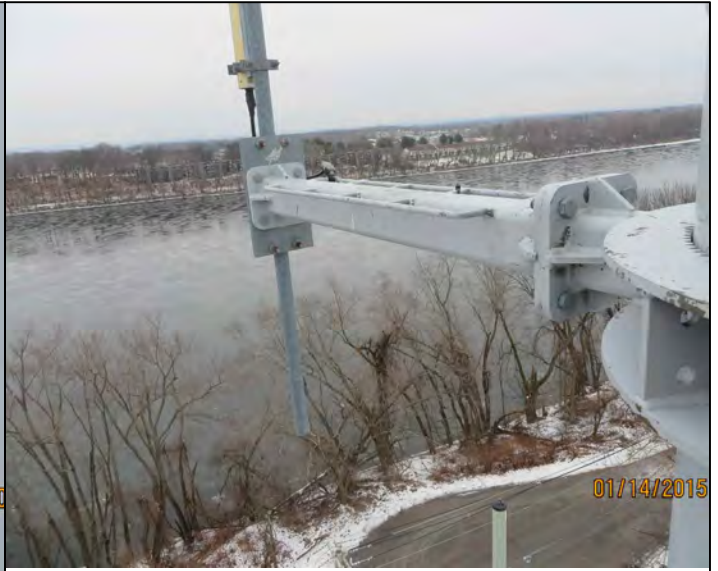
Photo From Tower
