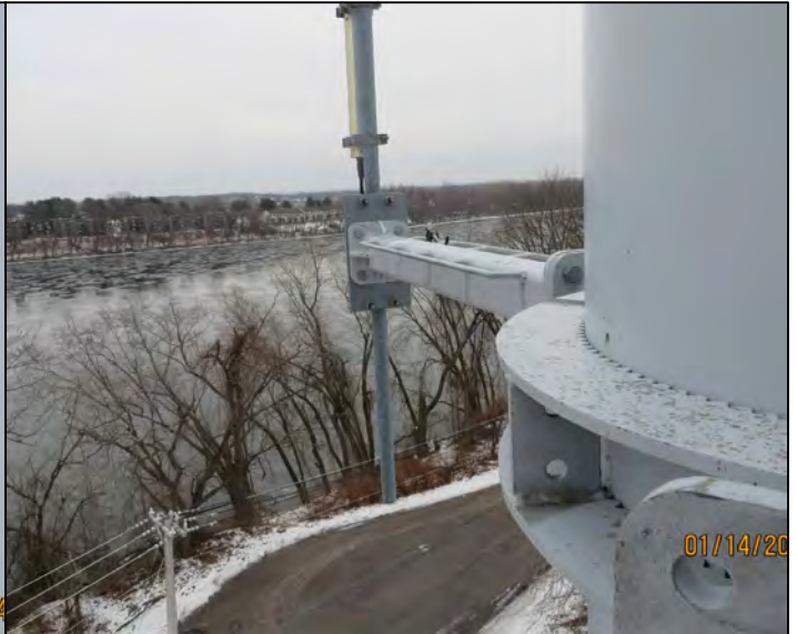
Photo From Tower
