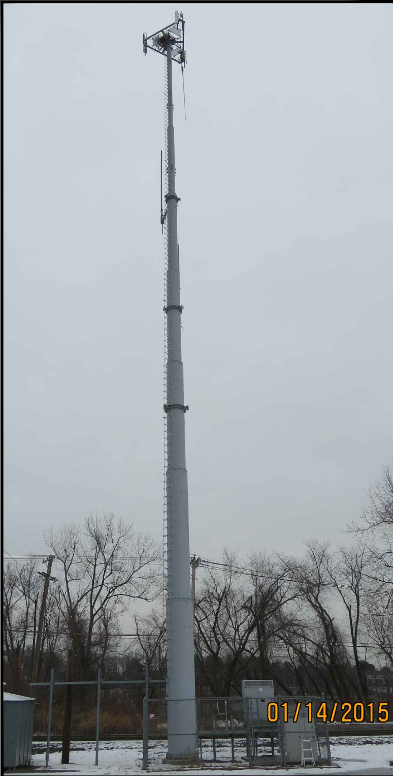
TOWER ELEVATION PHOTO
