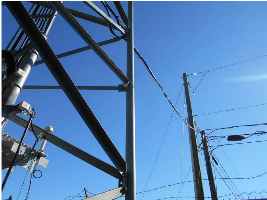
Photos of unlabeled feed lines on tower.
