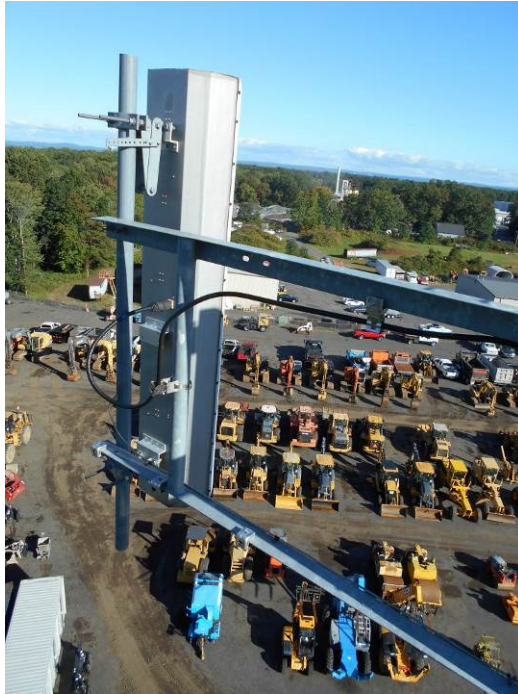
Additional photos of Verizon's typical existing equipment and mounts at 90.8'.
