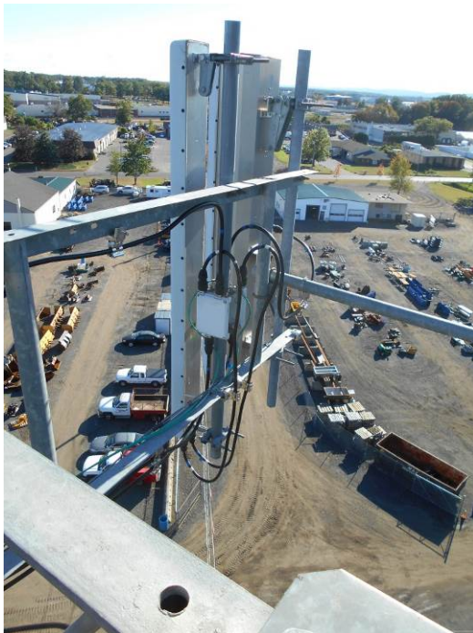
Additional photos of Verizon's typical existing equipment and mounts at 90.8'.
