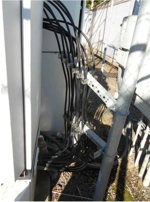
Photos of AT&T's existing feed lines and ground bar at cabinet.
