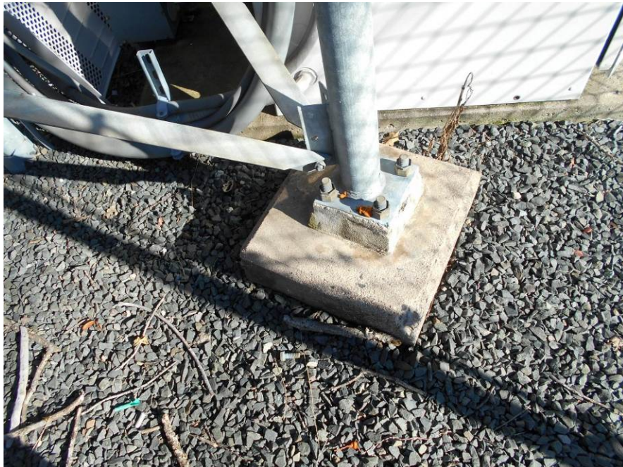
Photos of typical existing base foundations.
