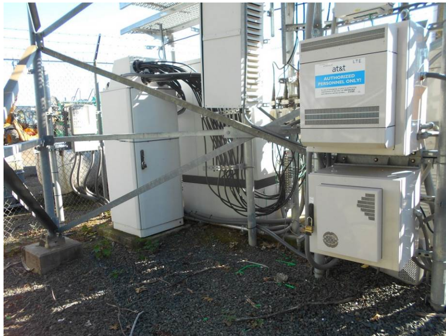
Photos of AT&T's existing feed lines and ground bar at cabinet.
