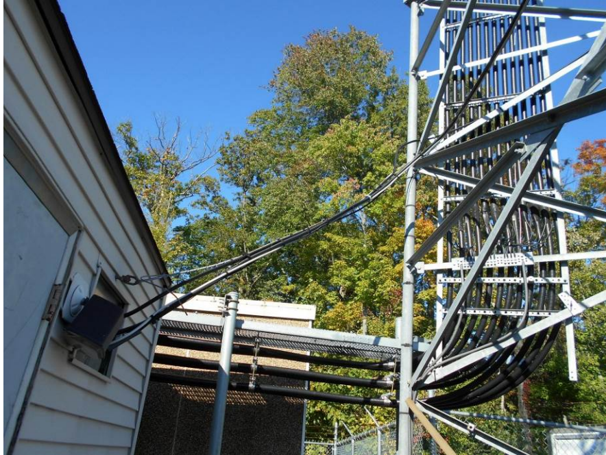
Photos of unlabeled feed lines on tower.
