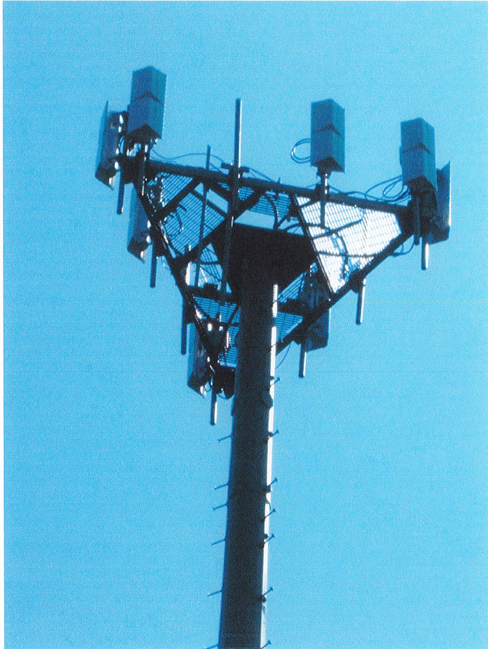
Photo showing existing antennas on 100' monopole tower located in Windsor, Connecticut.
