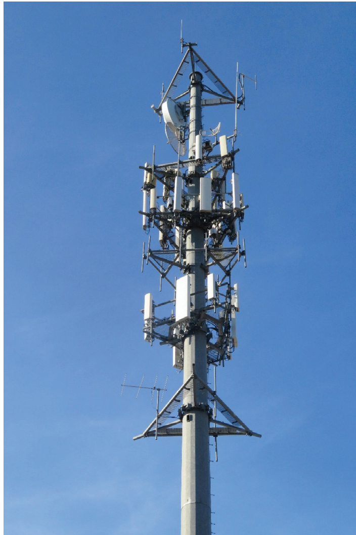
Photo 1: Photo illustrating the Monopole with Appurtenances shown.
