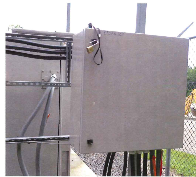
4 EXIST FIBER DISTRIBUTION BOX A-3 SCALE: NTS
