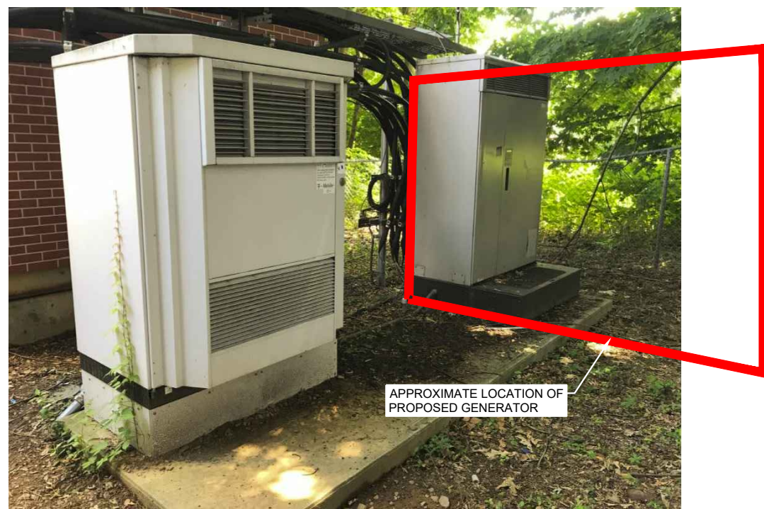
SITE PHOTO DETAIL SCALE: NTS 2 A-6
