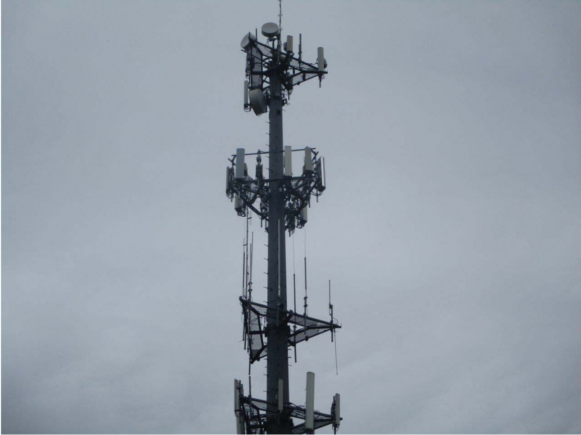
Photo 1: Photo illustrating the Tower with Appurtenances shown.
