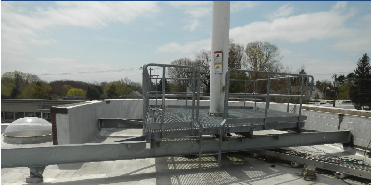
Existing Platform & Flagpole
