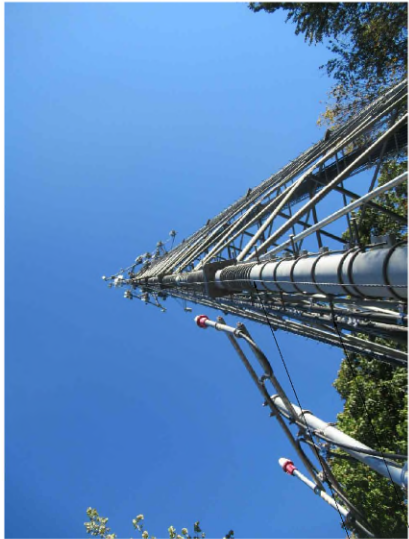
Existing Safety Climb
