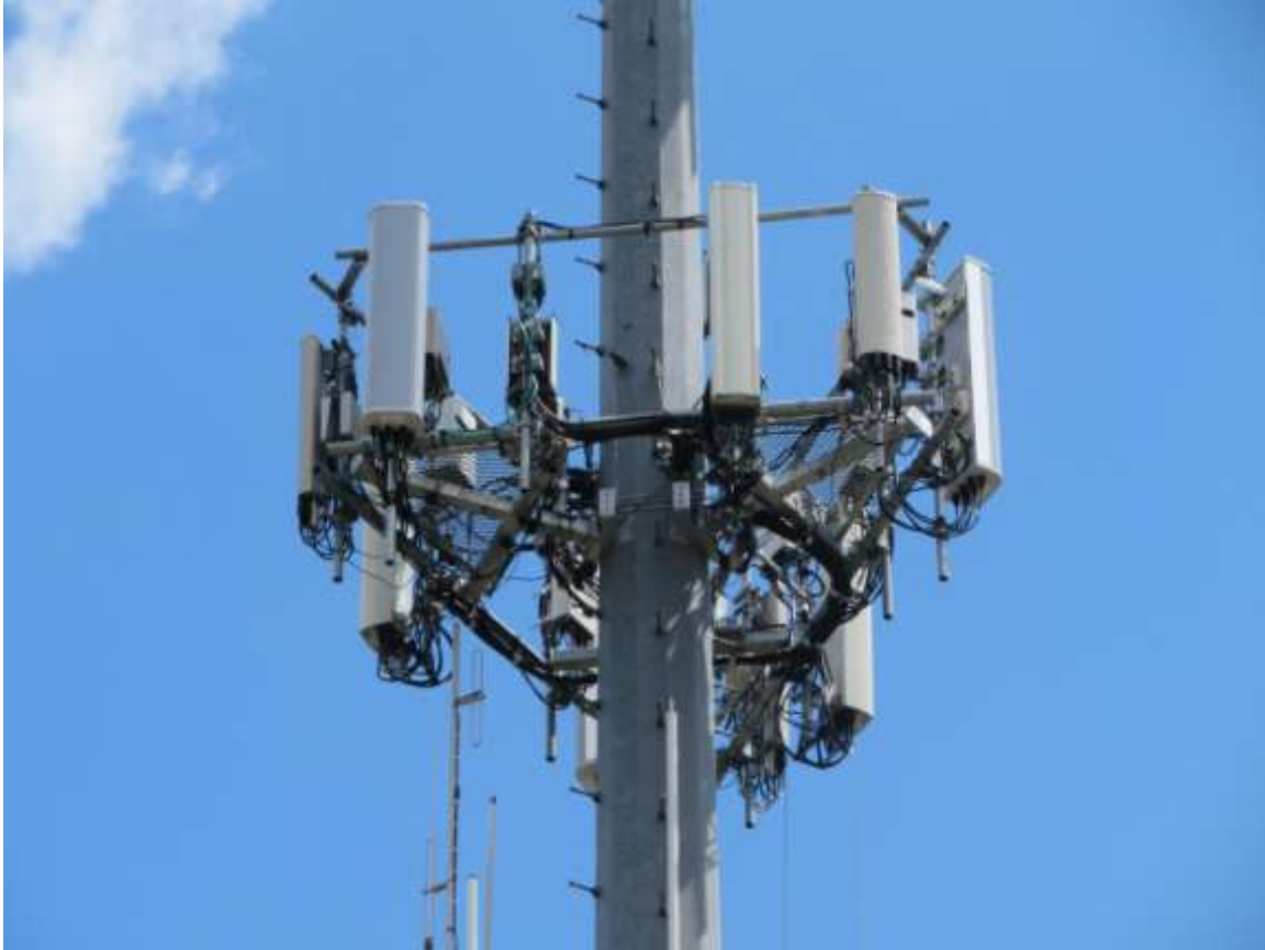
Photo 1: Photo illustrating the Tower with Appurtenances shown.
