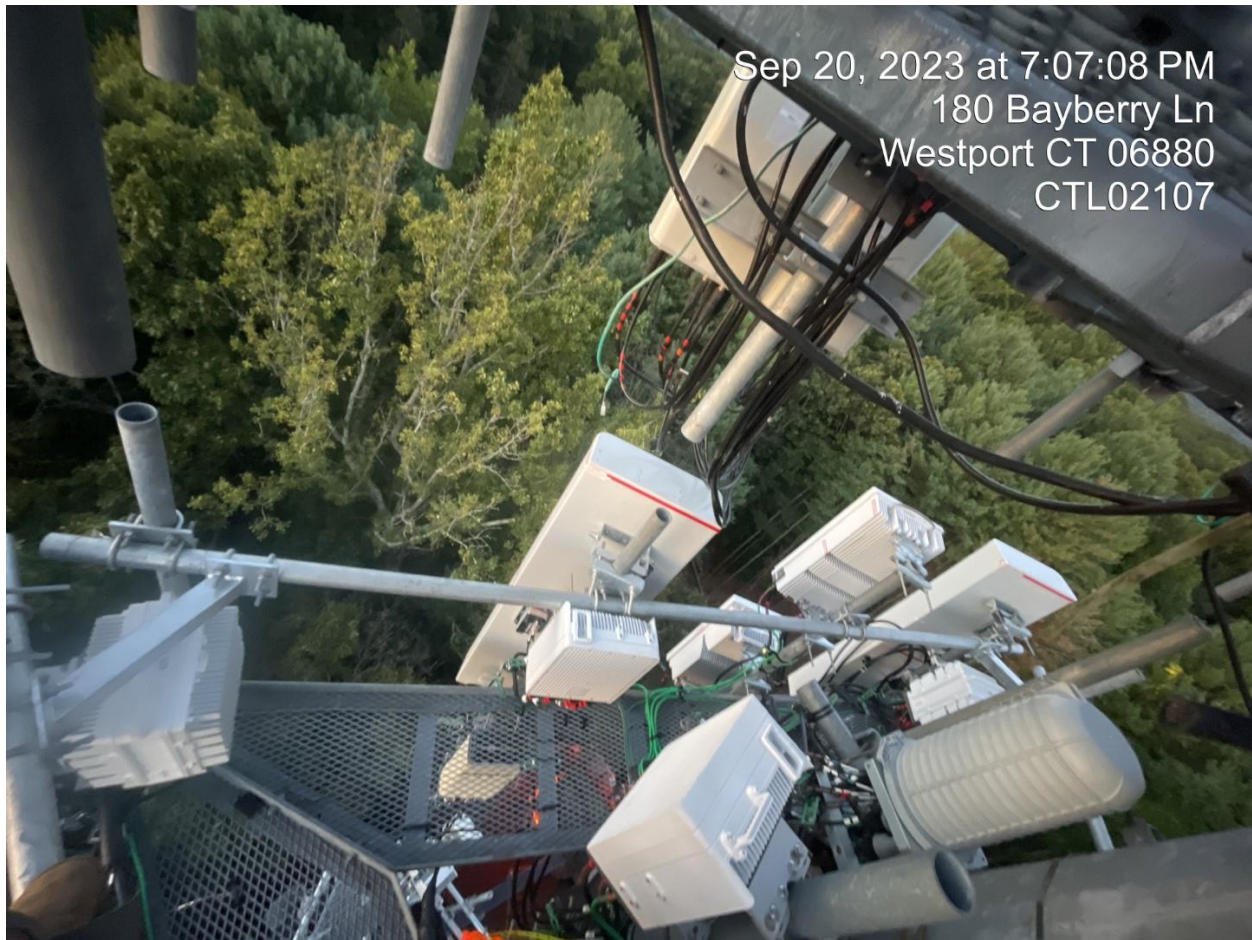
Photo - 1: Installation of Antennas and Equipment on Alpha Sector
