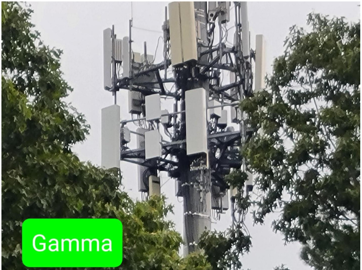
Photo - 6: Installation of Antennas and Equipment on Gamma Sector (From Ground)
