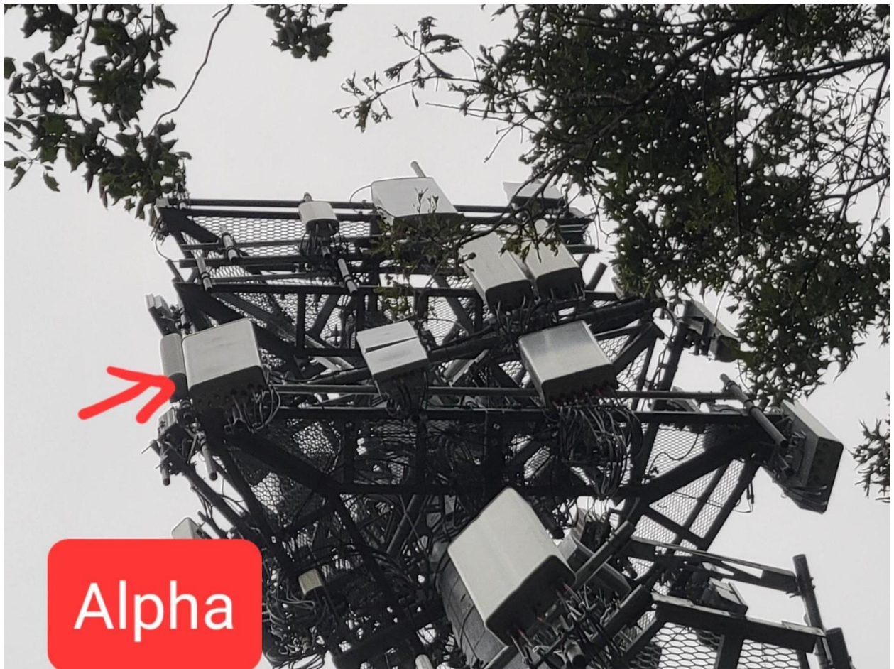
Photo - 4: Installation of Antennas and Equipment on Alpha Sector (From Ground)
