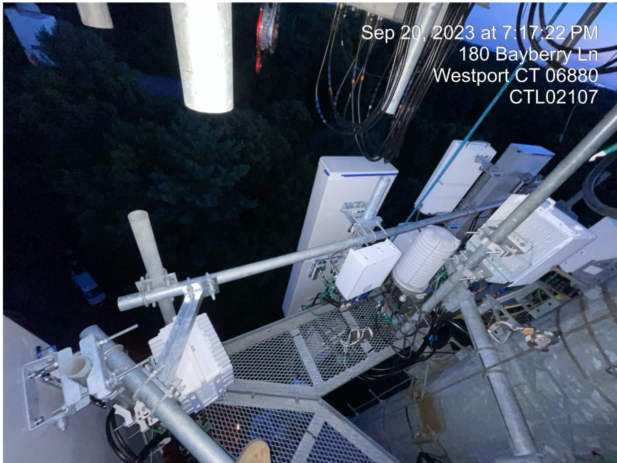
Photo - 2: Installation of Antennas and Equipment on Beta Sector
