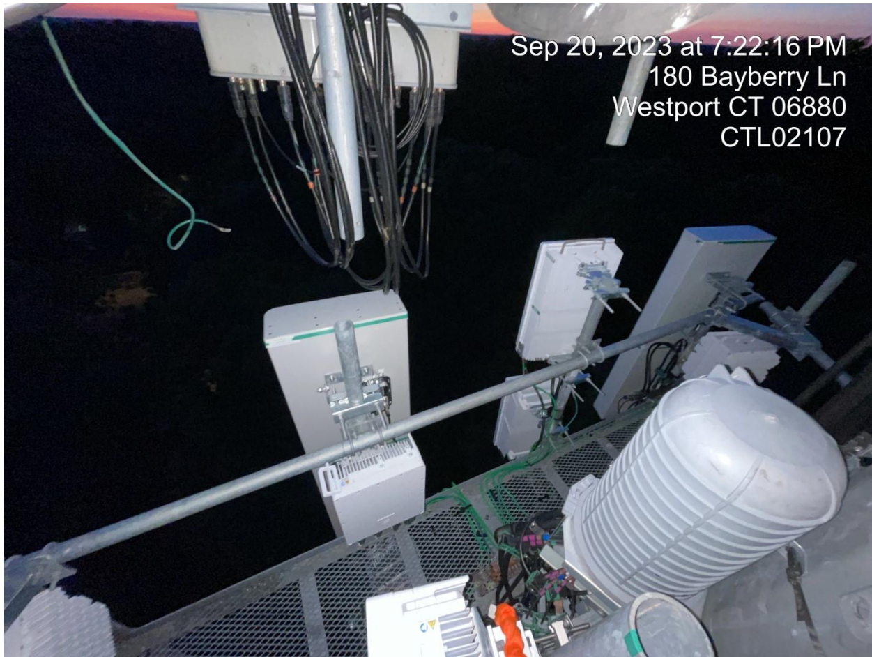
Photo - 3: Installation of Antennas and Equipment on Gamma Sector
